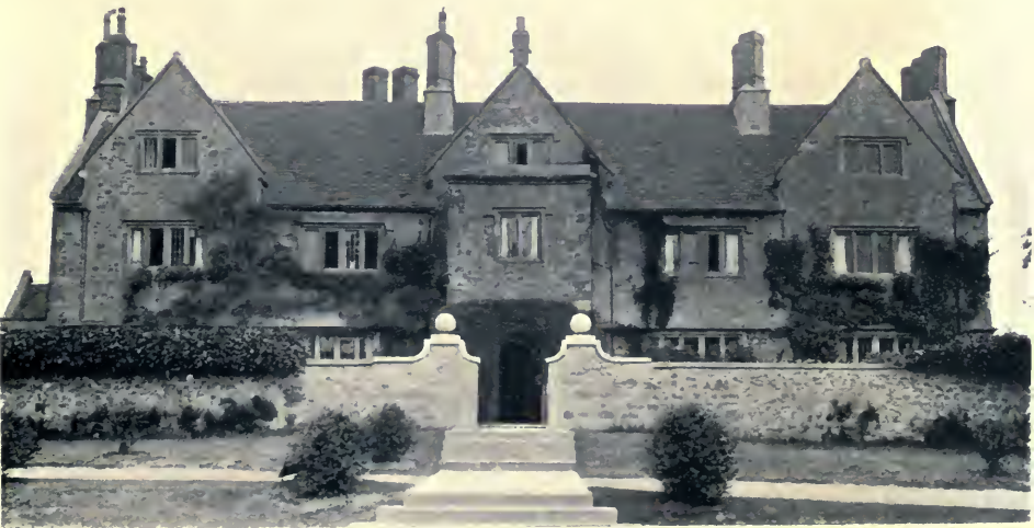
THE MANOR HOUSE, PURTON, SOUTH FRONT.
