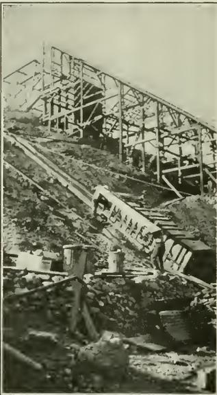
NEW MILL UNDER CONSTRUCTION BY SLATE RANGE MINERALS CO., INYO COUNTY, CAL. CUT SHOWS FLOTATION MACHINE ON SKIDS
