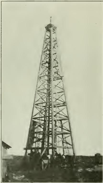
FIG. 4. DERRICK FOR ROTARY DRILLING 86 FT. IN HEIGHT
