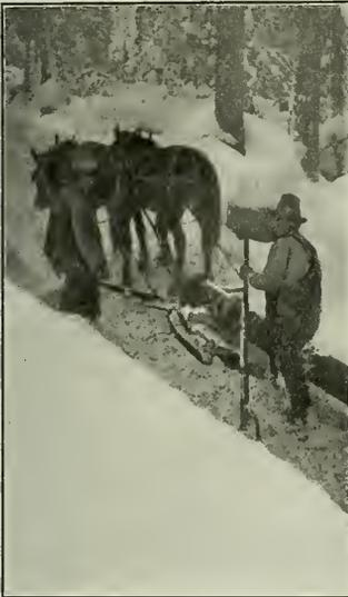
FIG. 1. HAULING 10-IN. PIPE UP 45 PER CENT GRADE.
