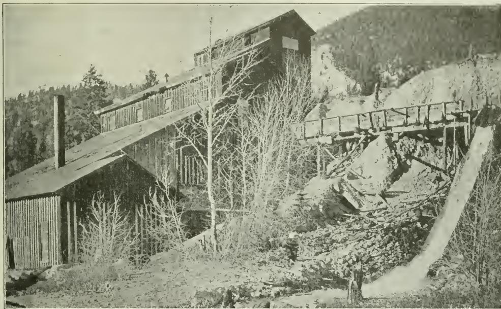
TRINIDAD MINING AND MILLING CO.'S MILL, FIVE MILES FROM R & S MINE. TEMPORARILY RENTED BY THE LATTER FOR CONCENTRATING ITS MOLYBDENITE ORES BY FLOTATION
