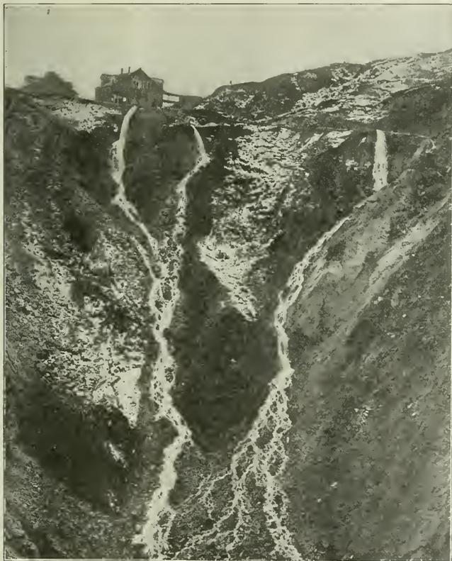
OPEN CUT OF HOMESTAKE MINE, LEAD, S. D., SHOWING STREAMS OF WATER BEING PUMPED INTO WORKINGS TO FLOOD BURNING STOPES
