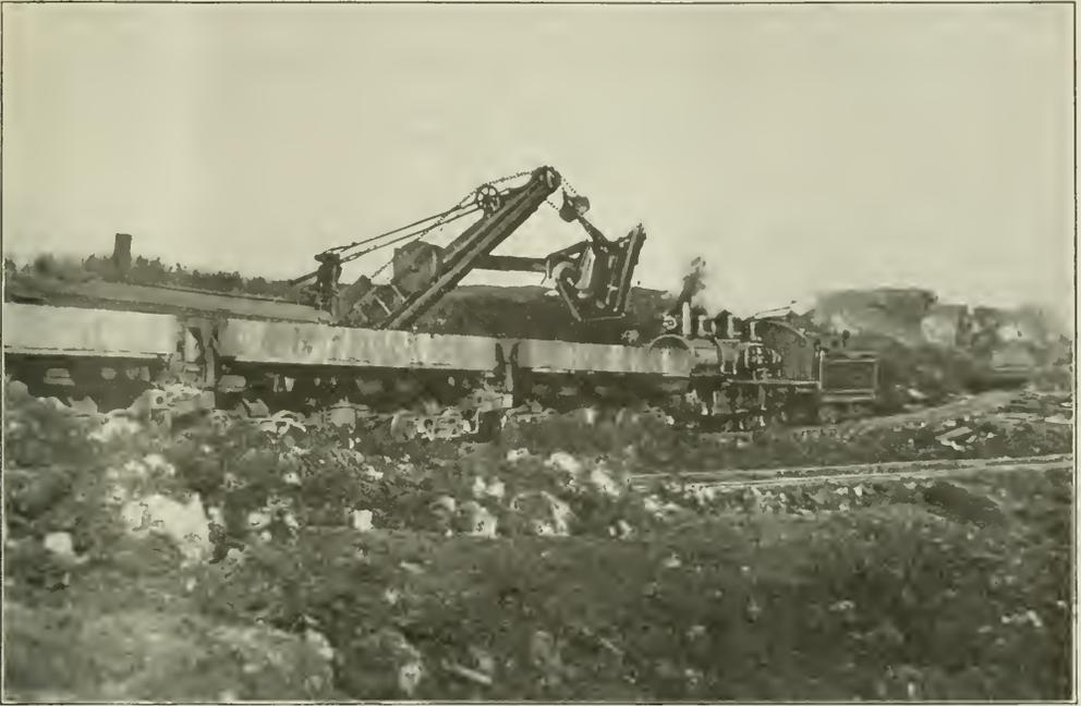
STEAM SHOVEL LOADING OVERBURDEN INTO 20-YD. AIR-STEEL AIR-DUMP CARS
