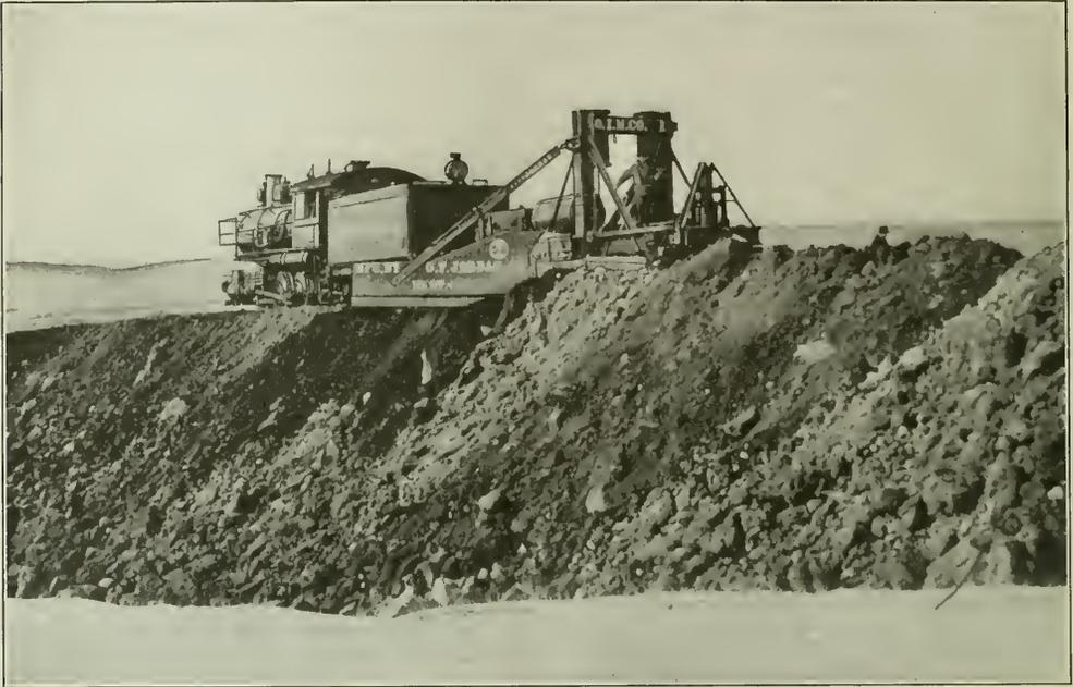
SPREADER BEING USED ON THE STRIPPING DUMP OF A MESABI RANGE OPEN-PIT MINE
