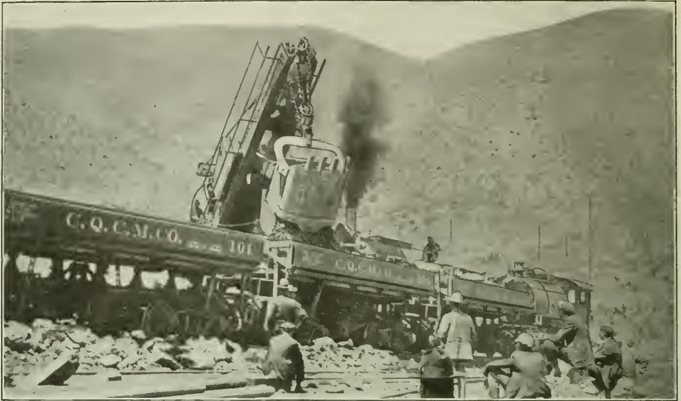
STRIPPING OPERATIONS OF COPPER QUEEN CONSOLIDATED MINING COMPANY AT BISBEE, ARIZONA. STEAM SHOVEL LOADING INTO 20-YD. AUTOMATIC AIR-DUMP CARS
