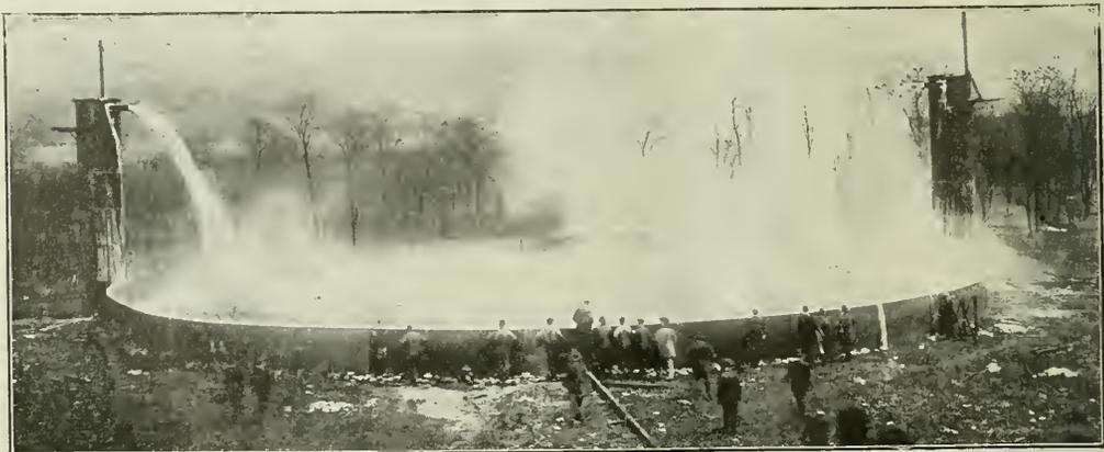
FIRE EXTINGUISHED WITHIN FORTY-EIGHT SECONDS AFTER THE APPLICATION OF CARBONIC-ACID GAS BUBBLES
