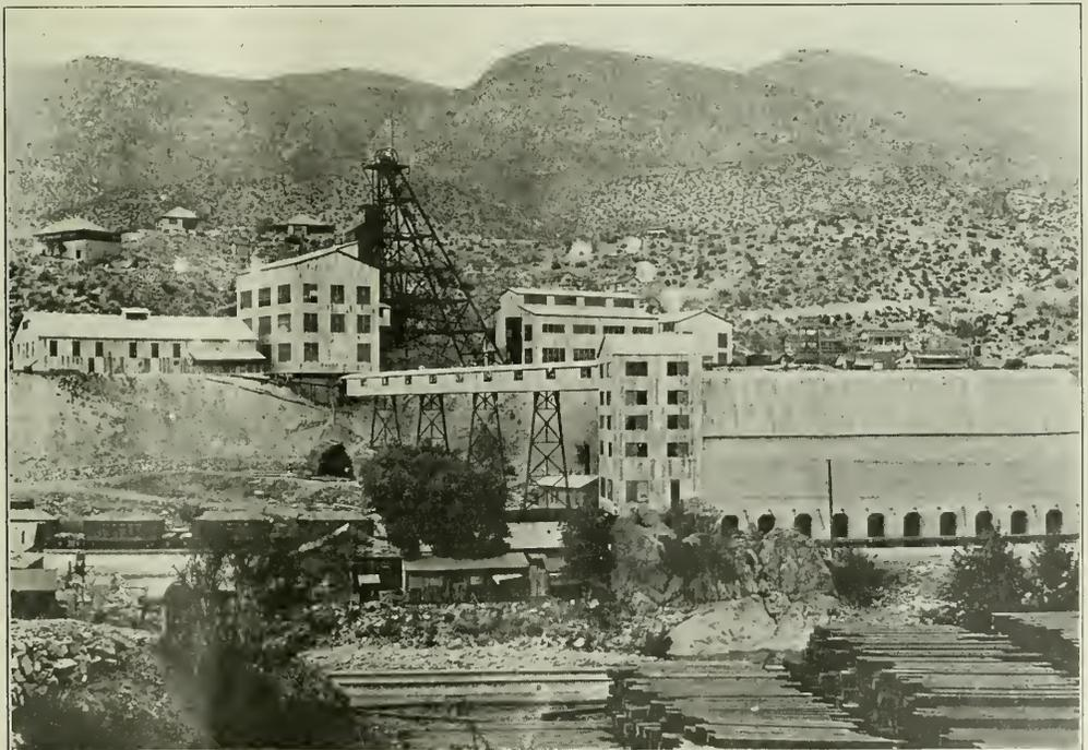
COARSE-CRUSHING PLANT, HEADFRAME, HOIST HOUSE AND MACHINE SHOP AT ARIZONA HERCULES
