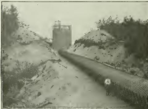
SURGE TANK IN COURSE OF CONSTRUCTION AND 84-IN. WOOD PIPE LINE, McCLURE PLANT
