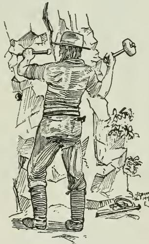
FIG. 2. MINER WITH SINGLE-JACK AND STEEL
