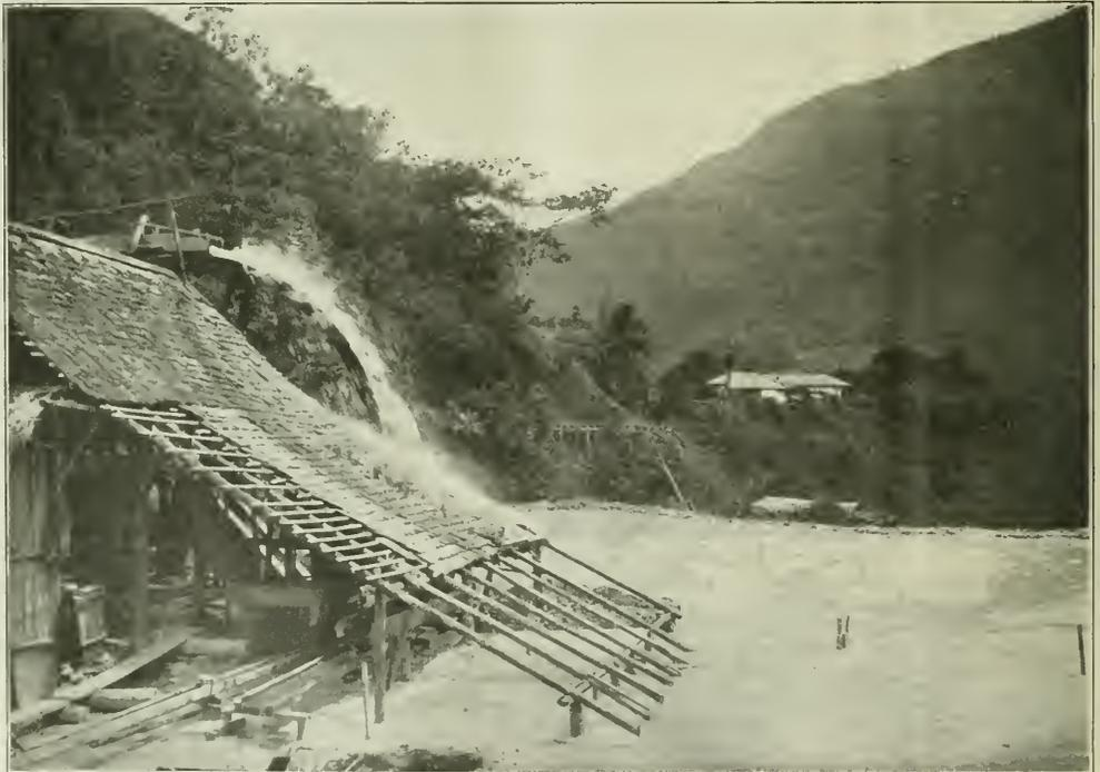
WOODEN STAMP MILL AND TAILINGS POND AT EL RECREO MINE. OWNER'S HOUSE IS SHOWN IN THE BACKGROUND, AND BELOW THAT CAN BE SEEN THE ROOF OF A SECOND WOODEN MILL.
