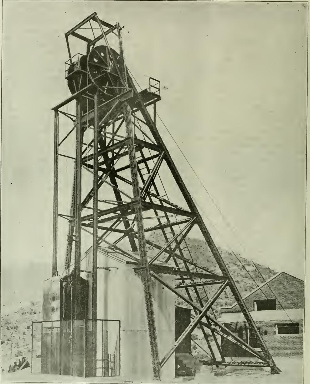
NO. 4 SHAFT AT RAY CONSOLIDATED, USED EXCLUSIVELY FOR HOISTING AND LOWERING MEN AND CARRYING POWER LINES
