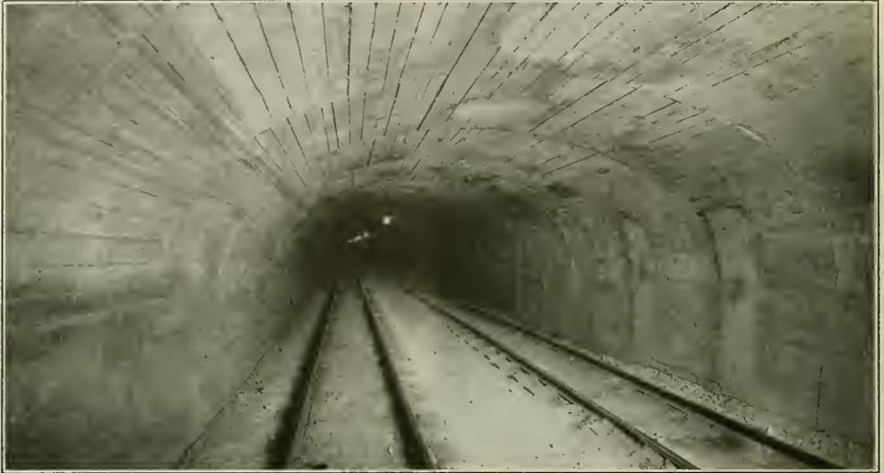
REINFORCED-CONCRETE SUPPORT OF DRIFT, NO. 3 LEVEL, RAY CONSOLIDATED COPPER CO., RAY, ARIZ.
