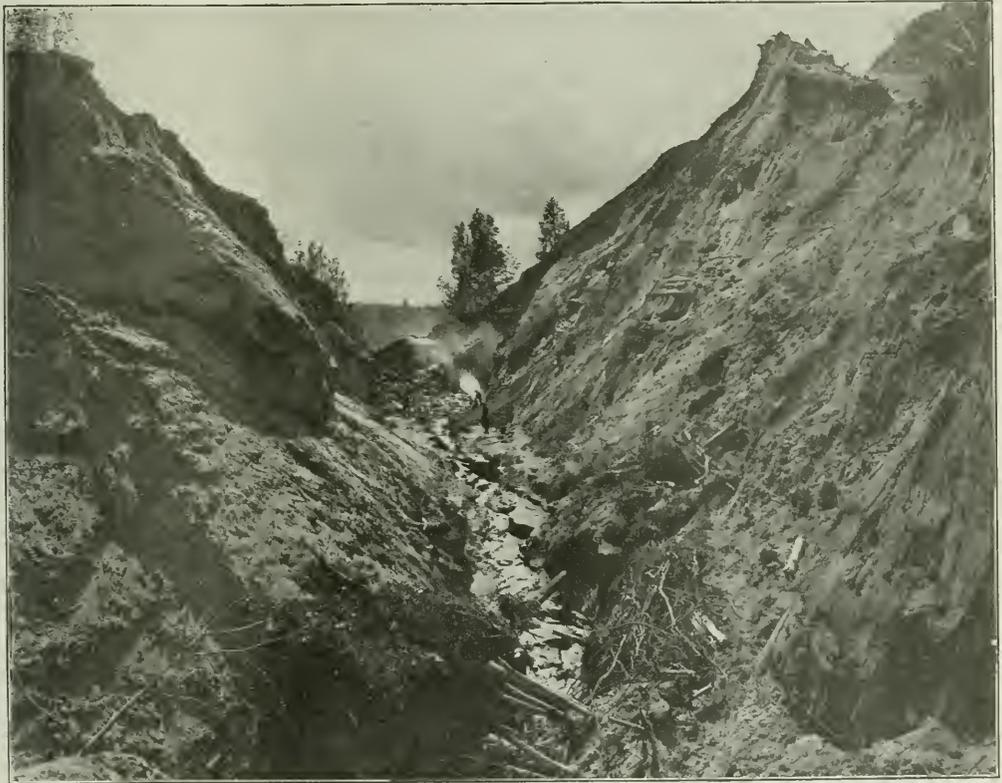
HYDRAULICKING THROUGH A HILL FOR THE PIPE LINE OF THE McCLURE PLANT
