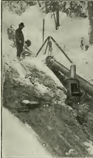
FIG. 2. LOWERING PIPE INTO A TUNNEL.
