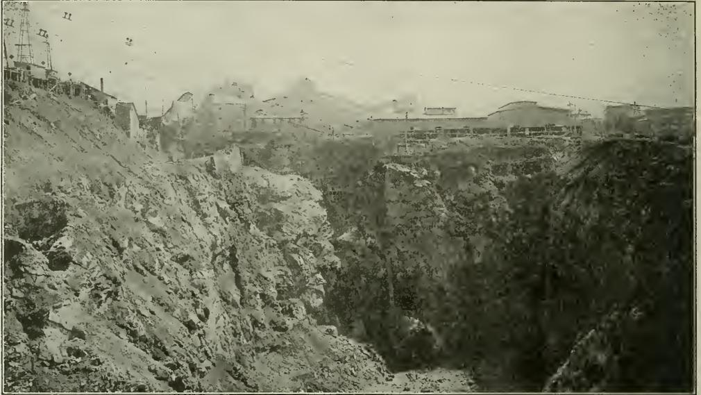
VIEW OF THE MINING PIT OR GLORY HOLE. THIS PIT IS ABOUT 300 FT. DEEP. SOME IDEA OF THE DEPTH CAN BE JUDGED BY THE SIZE OF THE MAN AT THE BOTTOM.
