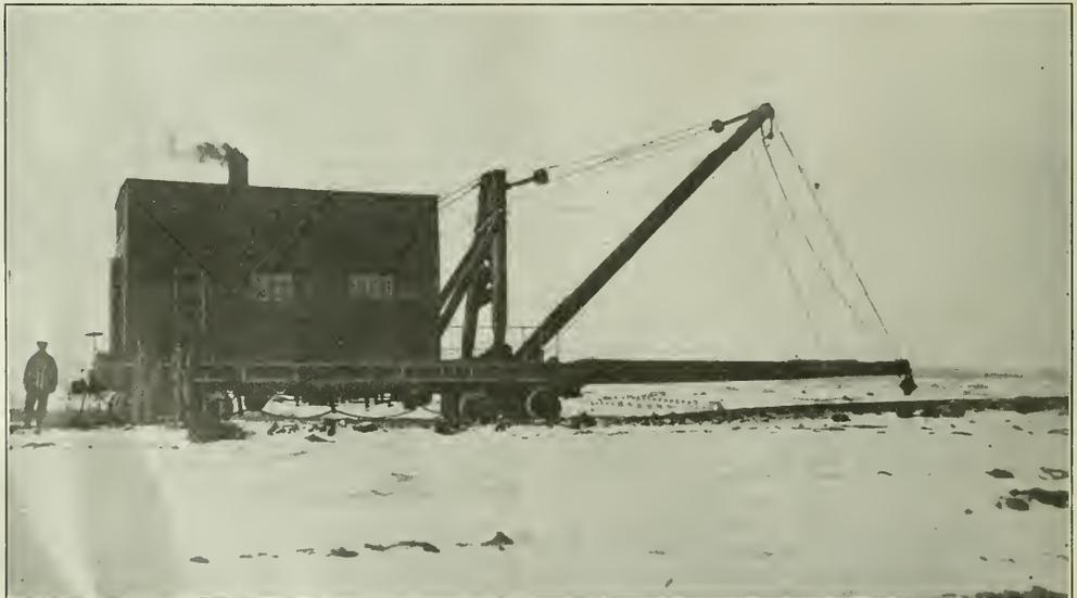
MECHANICAL TRACK SHIFTER USED IN MOVING TRACKS ON STRIPPING DUMPS
