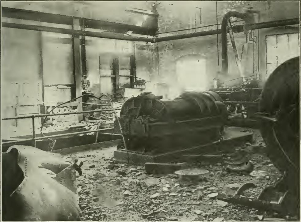
WRECK OF ENGINE ROOM CAUSED BY EXPLOSION OF GAS IN AIR-BLAST PIPE
