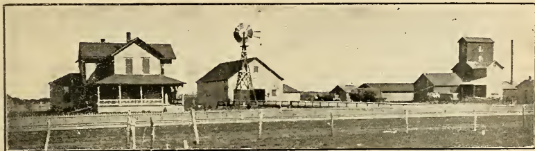
MR. HORACE ADAMS'S RESIDENCE AND ELEVATOR, Maple Hill.
