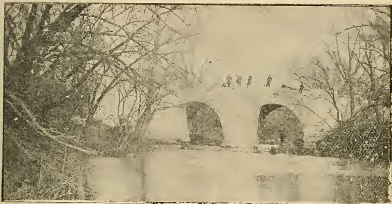
DOUBLE ARCH BRIDGE—FOUR MILES SOUTH-WEST OF ALMA
