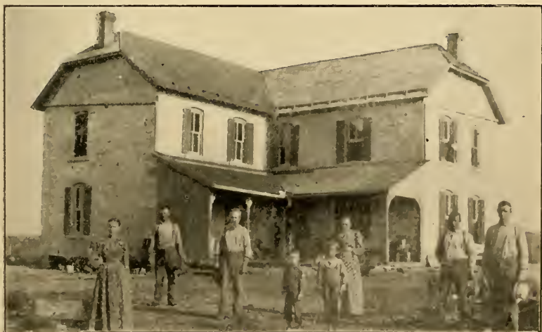
RESIDENCE OF MR. ALBERT DIEBALL, NEAR ALMA, 1901.
