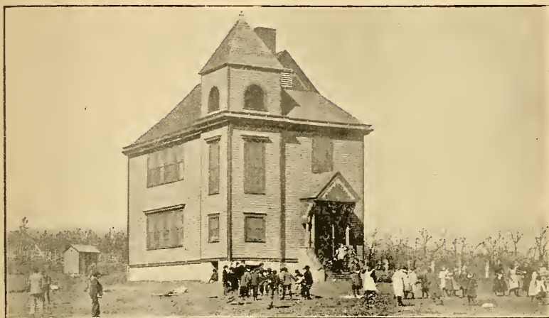
SCHOOL-HOUSE AT MCFARLAND.
