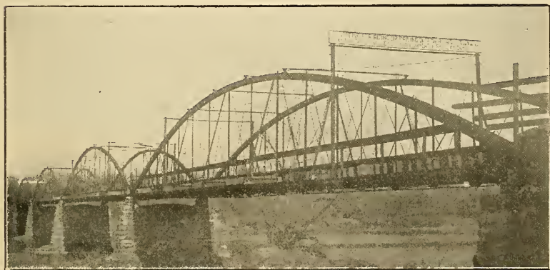
ST. MARY'S BRIDGE.
