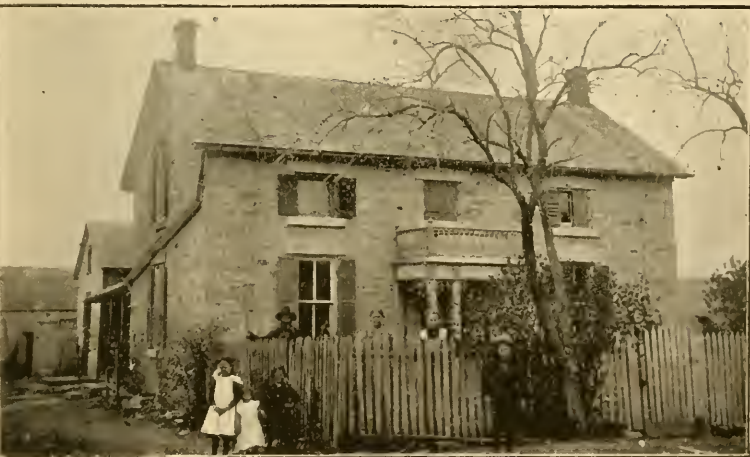
RESIDENCE OF MR. CHAS. ZECKER, on West Branch.
