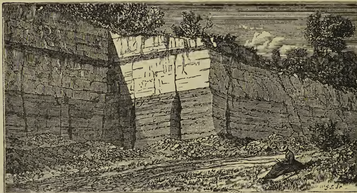
Fig. 33. Section at Snowdown, Chard, showing Upper Greensand, Lower Chalk, and Chloritic Marl.
