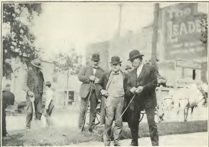
Surveying at Franklin Circle for three-cent fare line
