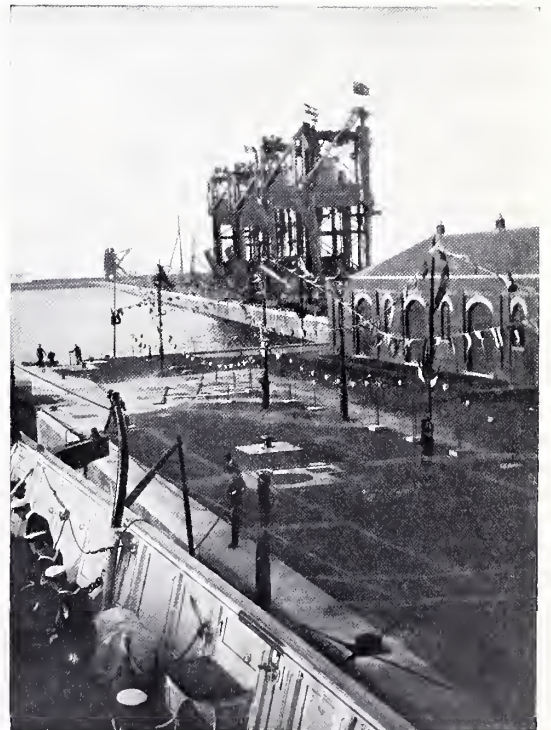
The Opening of the Alexandra Dock, Cardiff, 1907.
