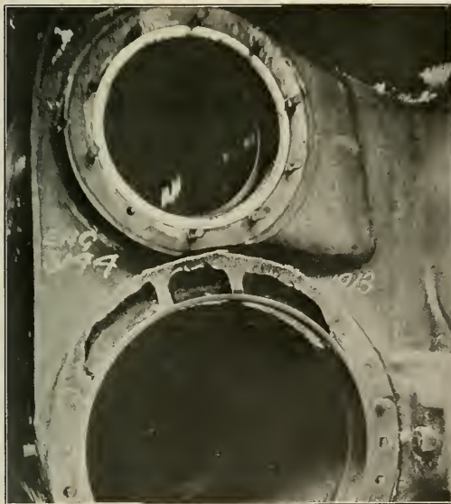
Fig. 8—Broken Cylinder Repaired by Arc Welding
