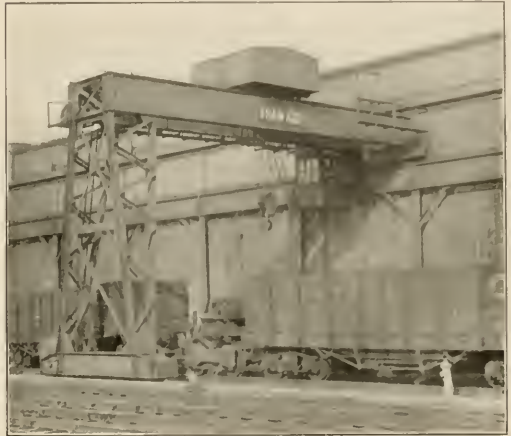
Gantry Crane over Heavy Material Storage
