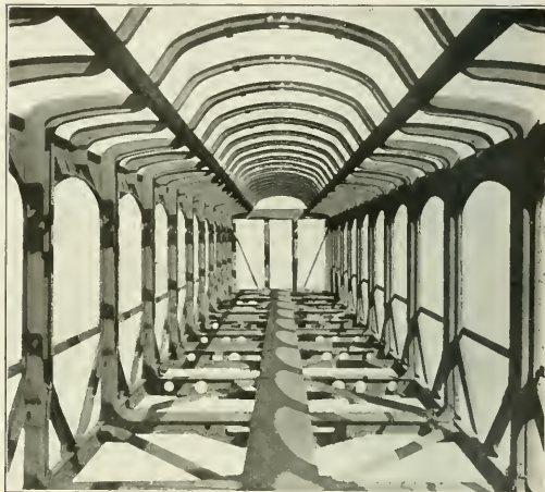
Interior View of the Completed Framing; Erie Suburban Cars
