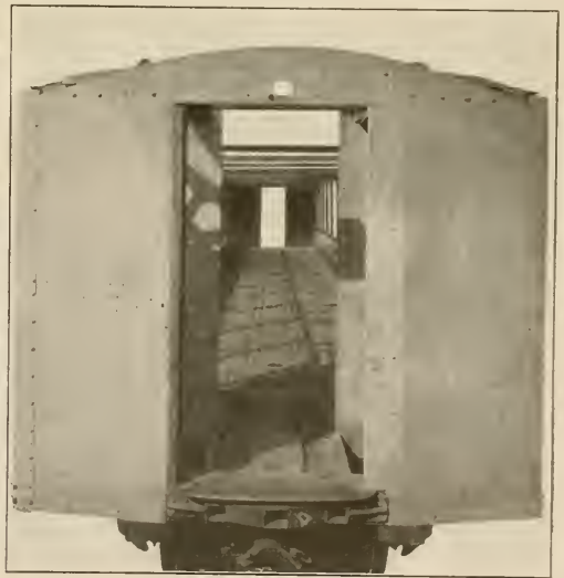
An End View of the Steel Work
