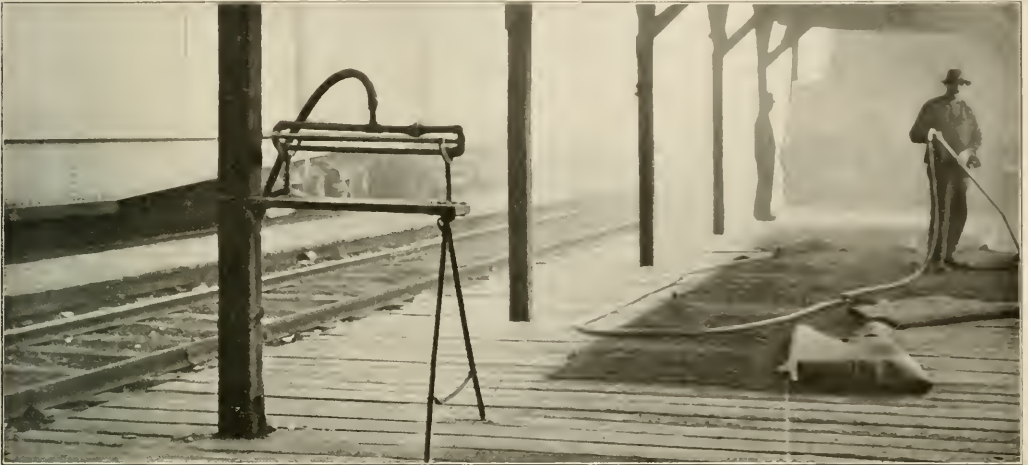
Apparatus Used for Cleaning Carpets by Compressed Air on the Chicago & Western Indiana
