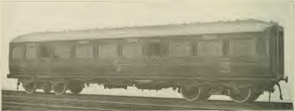
All-Steel Kitchen Car Used on the East Coast Route in England
