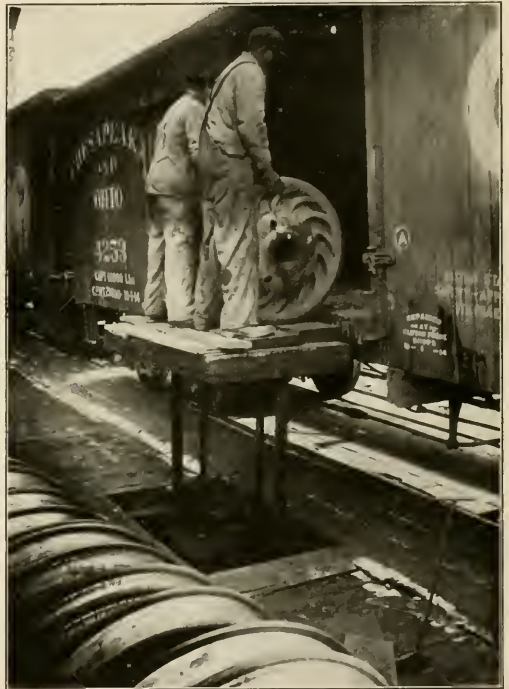
Hoist for Loading Scrap Wheels
