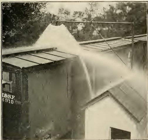
Testing Car Roofs for Leakage at the Topeka Shops of the Atchison, Topeka and Santa Fe
