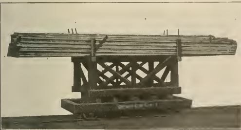
Fig. 6—Rotary Car for Transporting Repaired Tubes to the Erecting Shop
