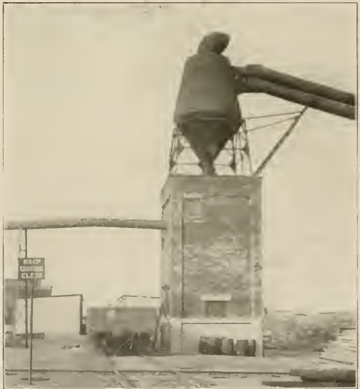
Sawdust House and Separator for Planing Mill
