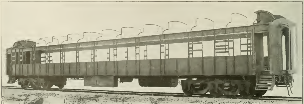
Steel Framing for a Car Which Has Wooden Sheathing
