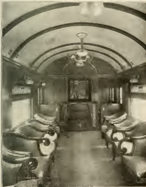
An Interior View of the Baggage-Buffer Car
