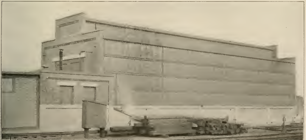
Sand Blast House; the Sides Are Enclosed with Continuous Operating Sash
