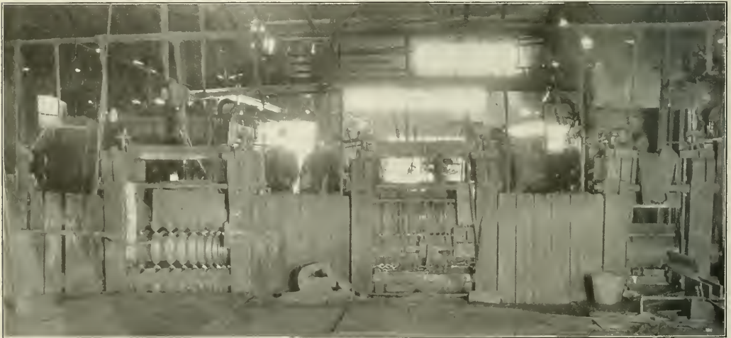
Fig. 5—Rear View of the Rolling Mill; Roughing Rolls on the Left
