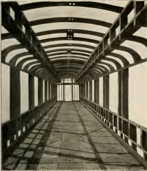
Framing of the Santa Fe Steel Passenger Cars
