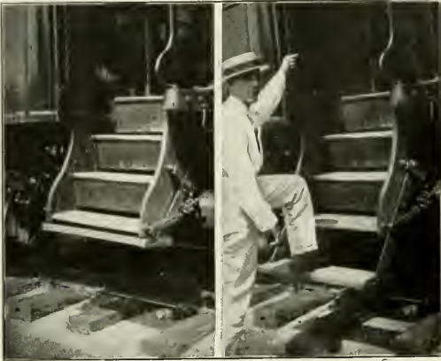
Adjustable Step in Raised and Lowered Positions
