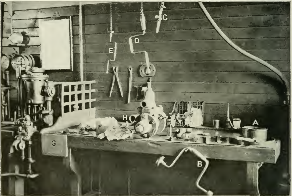
Arrangement of Bench for Cleaning Triple Valves
