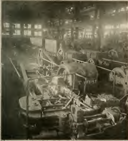
Rivet Heading Machine with Overhead Crane and Storage Bins in the Background
