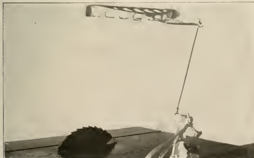
Fig. 3—Saw Guard Swung Back from the Table
