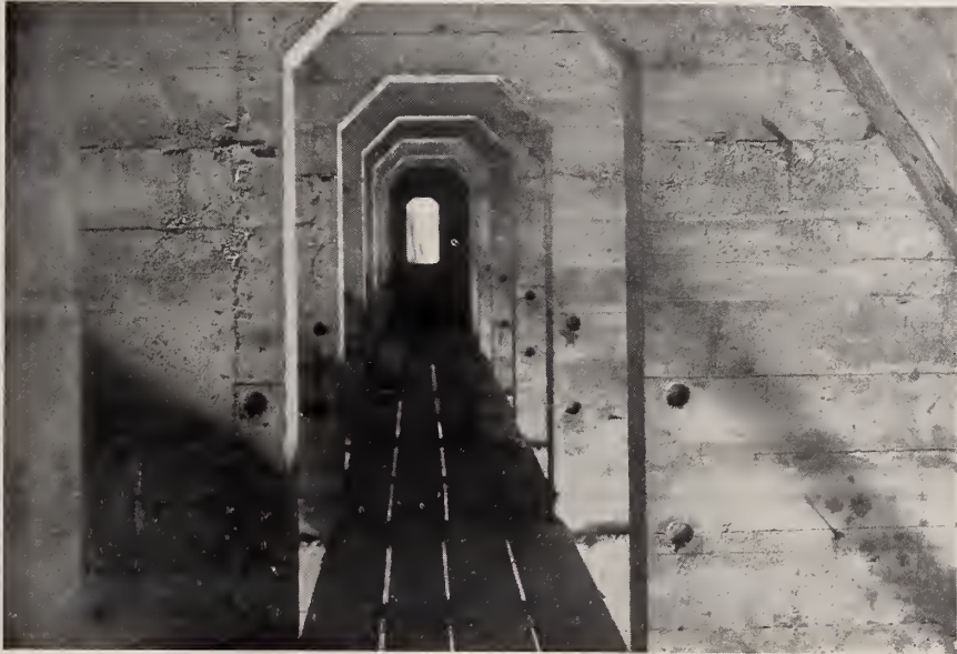
SCHUYLERVILLE DAM. View of interior.
