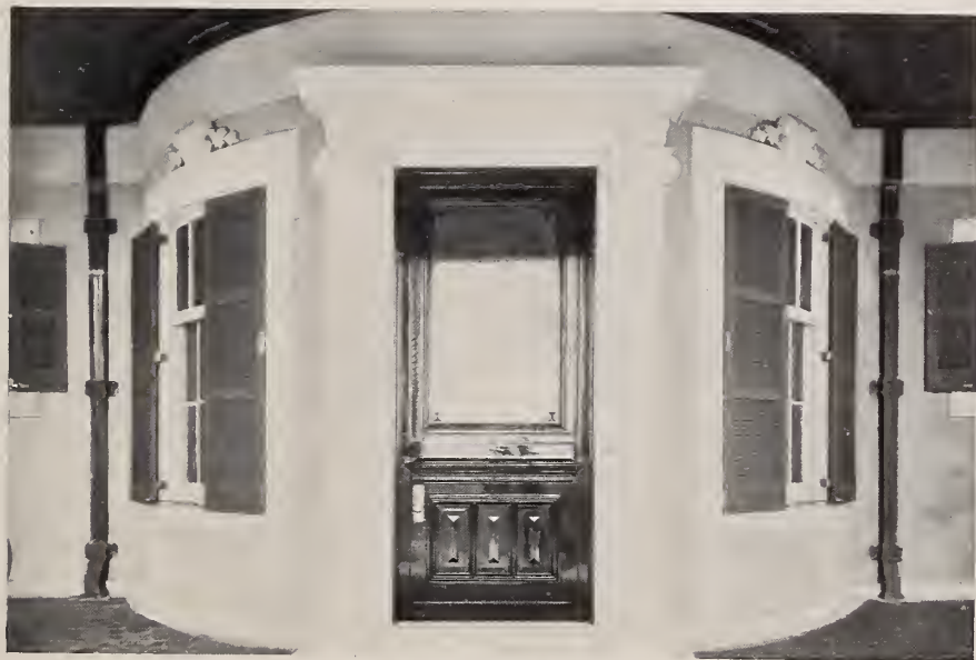
DETAIL OF ENTRANCE, SCRYMSER HOUSE, SEABRIGHT, N. J.
