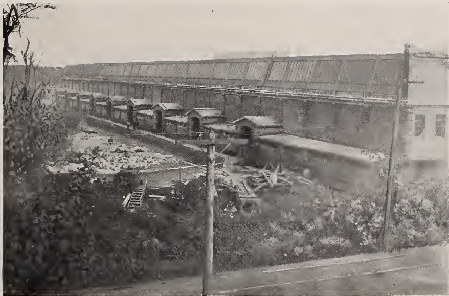
STOLLWERCK BROS. CHOCOLATE FACTORY, STAMFORD, CONN. The building is 500 feet long and 100 feet wide.
