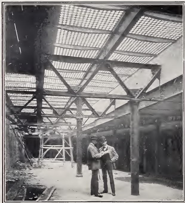
STEEL-CONCRETE VAULT LIGHTS AT 59TH STREET STATION, NEW YORK SUBWAY.
