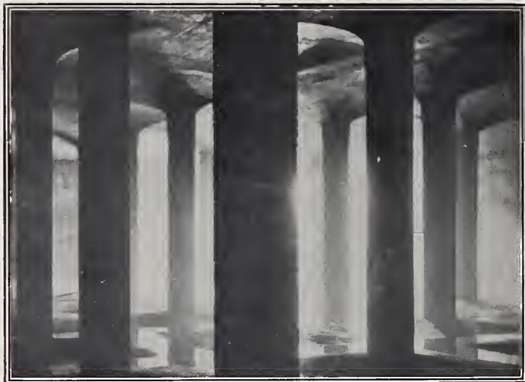
FILTRATION PLANT FOR ITHACA WATERWORKS CO., ITHACA, N. Y. Interior of Clear Water Basin.
