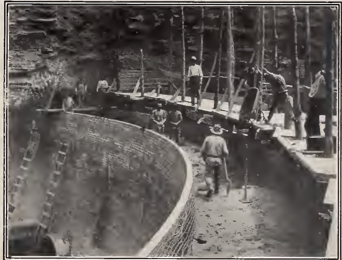
Showing method of construction.
