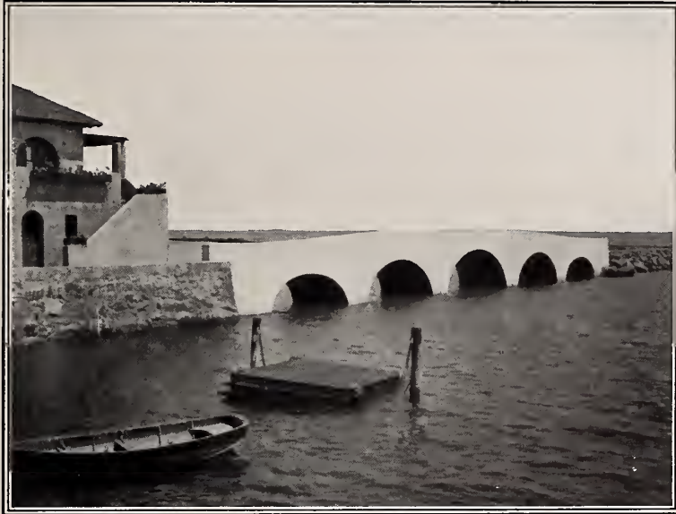
REINFORCED CONCRETE BRIDGE AT MAMARONECK, N. Y.
