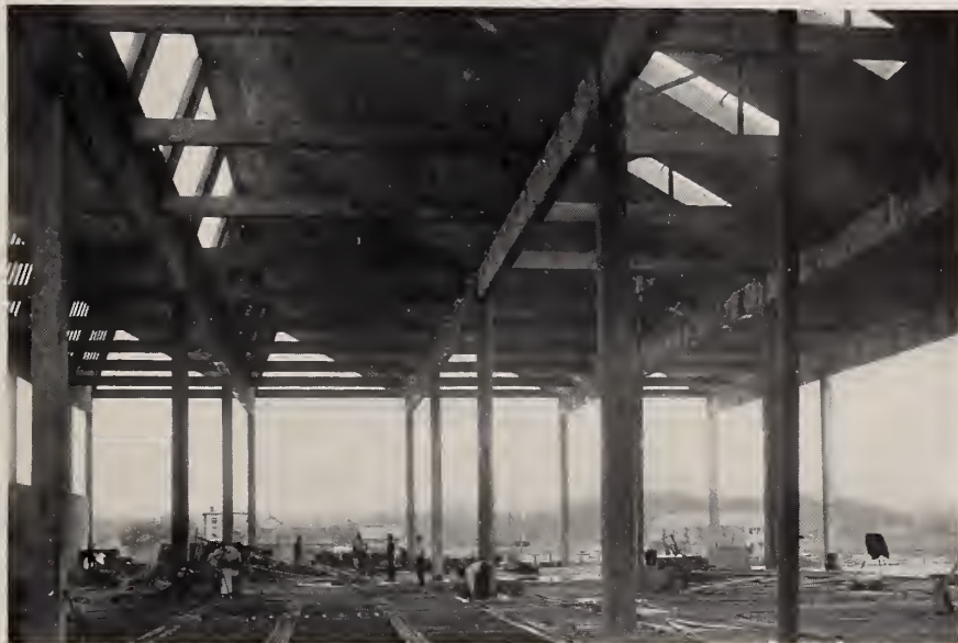
INTERIOR STOLLWERCK FACTORY. Showing saw-tooth on fifty foot span.
