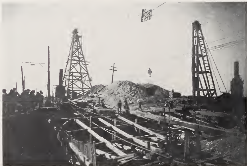
DERBY BRIDGE. Excavating for west abutment.
