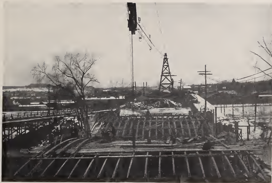
DERBY BRIDGE. Showing centering and reinforcement in place ready for concrete.
