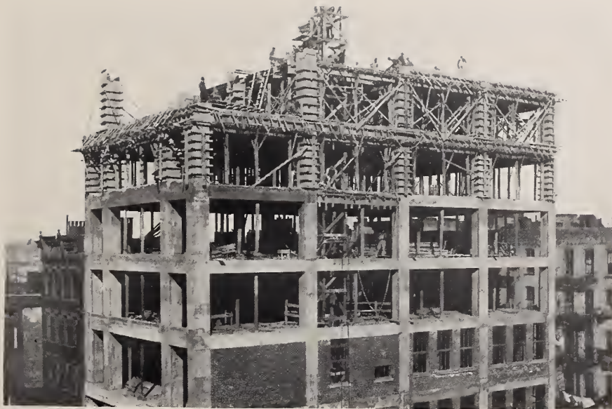
McNULTY BUILDING. Tenth floor finished and the roof forms being set.
