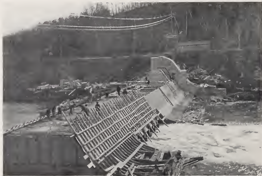
SCHUYLERVILLE DAM. Showing method of construction.
