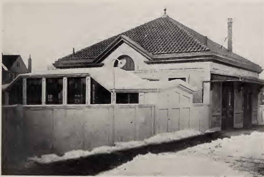
DETAIL OF BRIDGE AND WAITING ROOM OF NEWKIRK AVENUE STATION.
