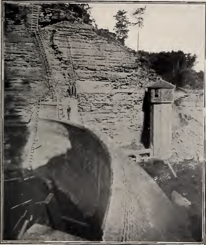
General View—showing Gate House and Intake Tower
