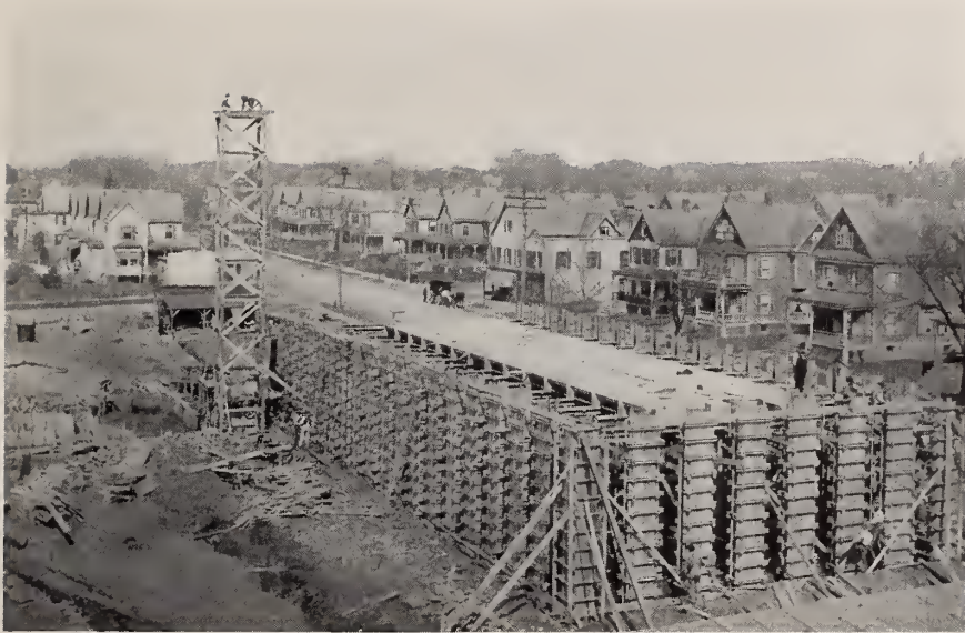
FACTORY, RUSHMORE DYNAMO WORKS, PLAINFIELD, NEW JERSEY. Showing methods of centering.
