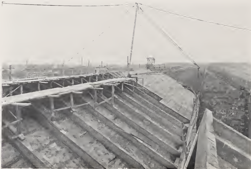
STOLLWERCK FACTORY. Showing hollow roof construction.
