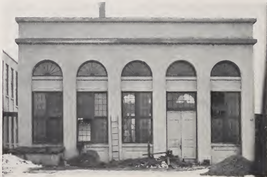
POWER HOUSE, RUSHMORE DYNAMO WORKS, PLAINFIELD, NEW JERSEY.
