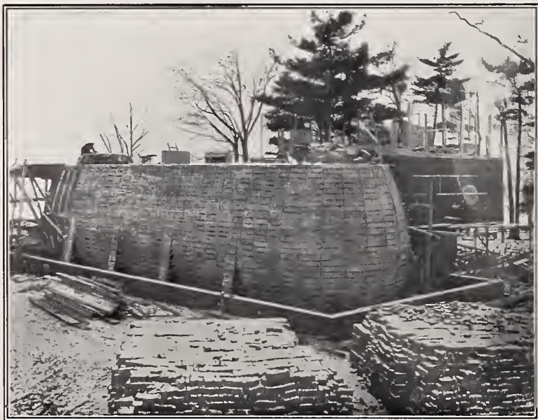
STEEL-CONCRETE MECHANICAL FILTER, CORNELL UNIVERSITY. General View—before construction of outside walls.
