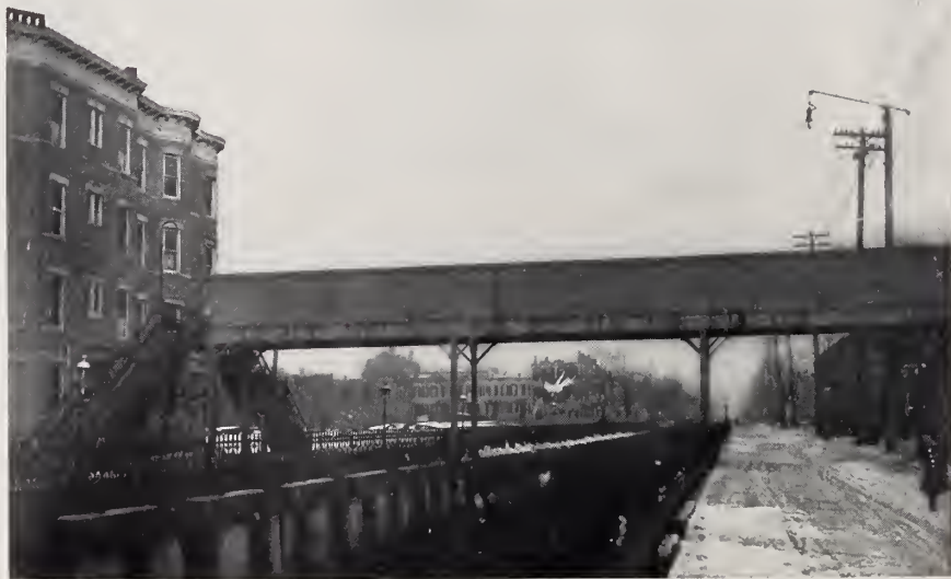
BRIDGE ON ATLANTIC AVENUE FOR LONG ISLAND RAILROAD CO.
