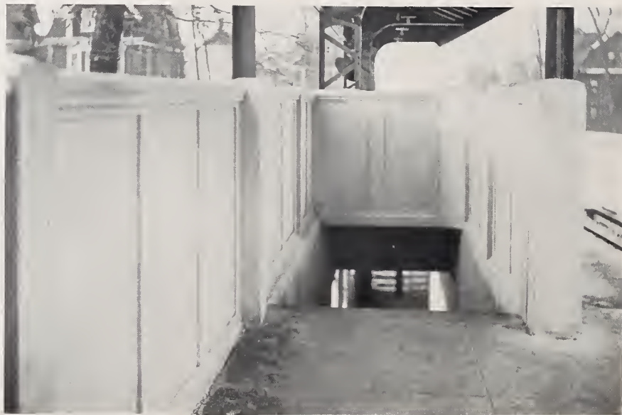
DETAIL OF FENCE ON AVENUE H STATION. This fence is molded in place and the panels are but 2\frac{1}{4} inches thick.
