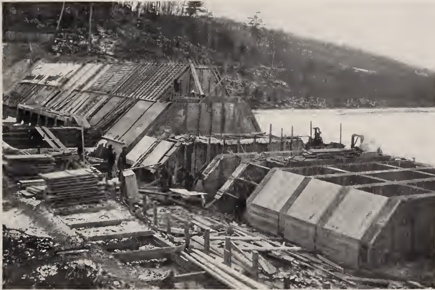
SCHUYLERVILLE DAM. Showing method of centering.
