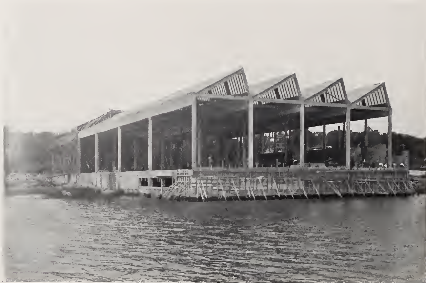
EXTERIOR OF STOLLWERCK FACTORY. Showing saw-tooth roof on fifty foot spans.
