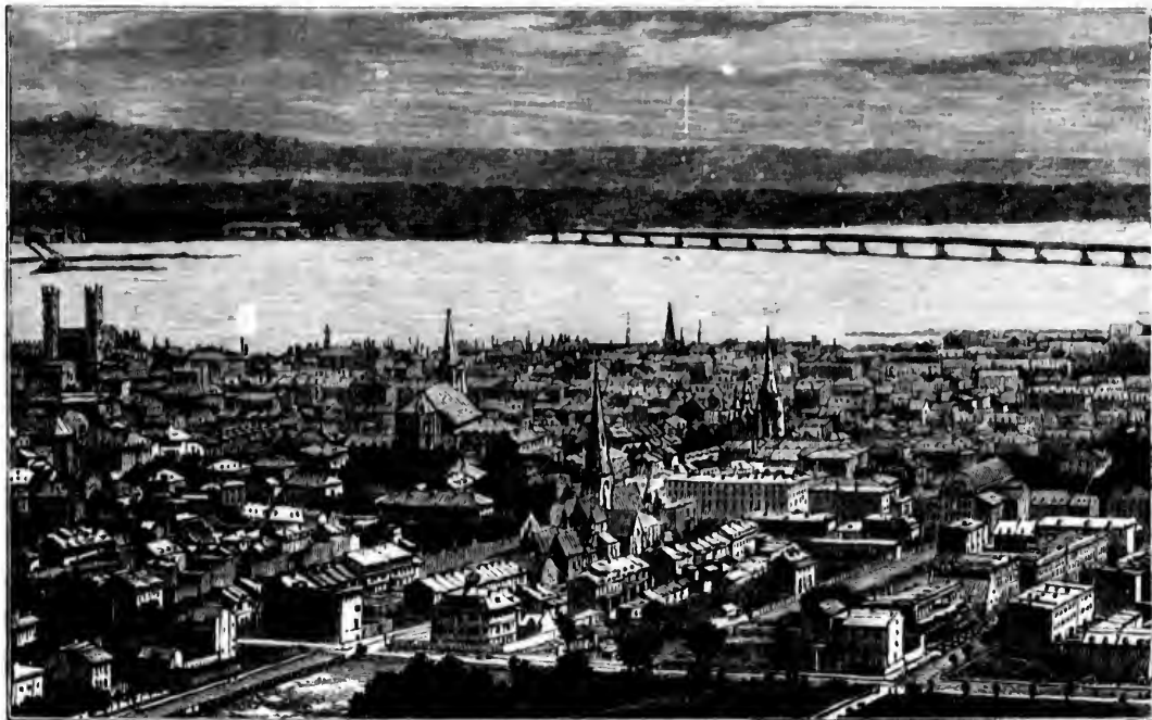
81. MONTREAL, AND VICTORIA BRIDGE ACROSS THE ST. LAWRENCE.
