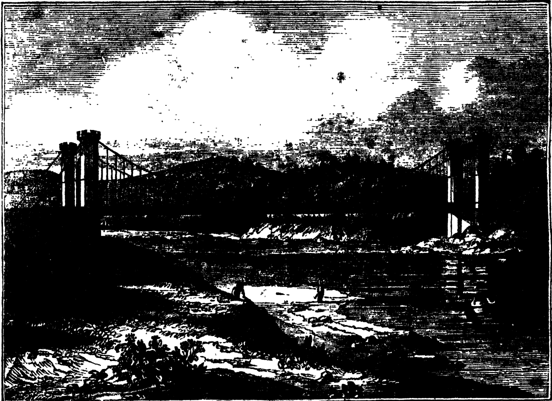
[Findhorn Suspension Bridge.]
