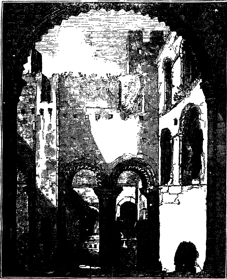
[Interior of the remains of the Upper Story of Rochester Castle.]
