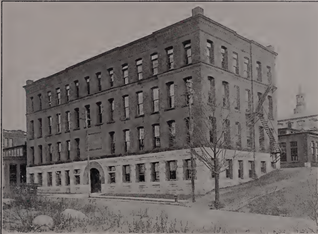
MECHANICAL ENGINEERING BUILDING
