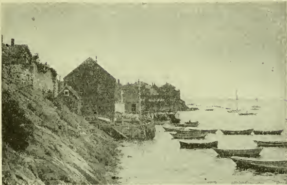
Quaint Old Houses Line Marblehead Shore
