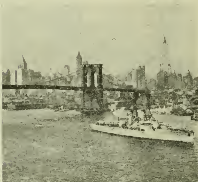
New York City and a Guardian Man-of-War Singer Building. Woolworth Building. Municipal Building.
