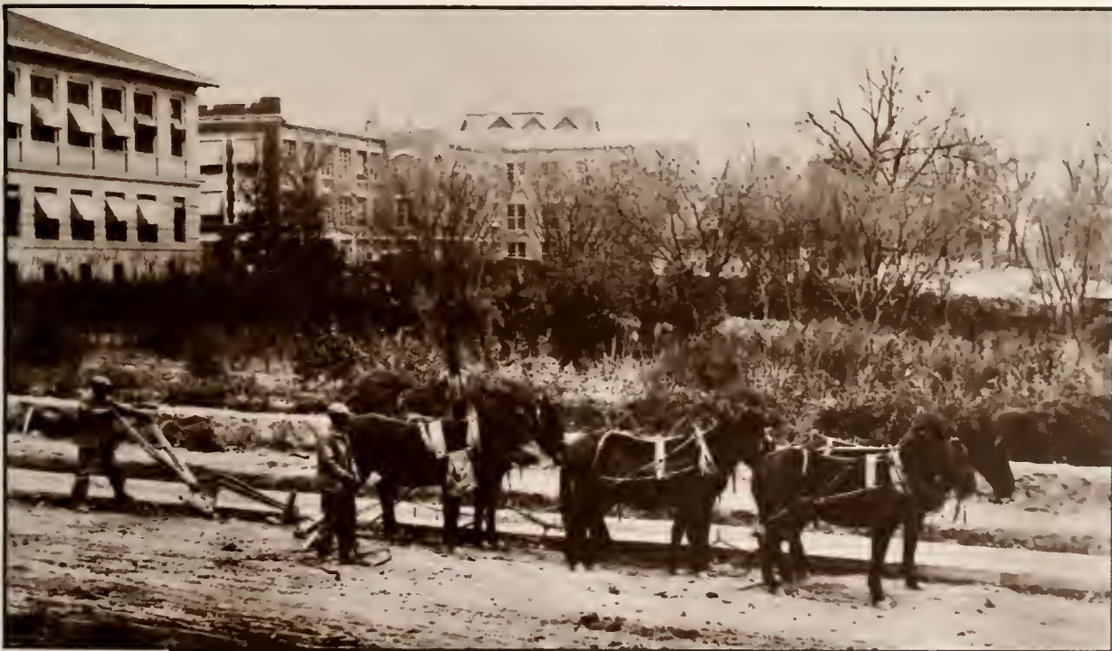
Construction of Columbia Street.
