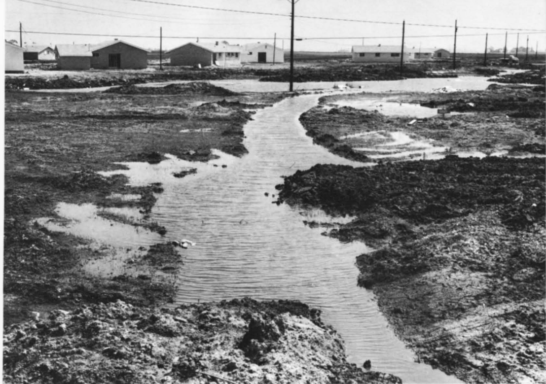
Poor drainage is manifest in this subdivision in Cook County in Illinois.
