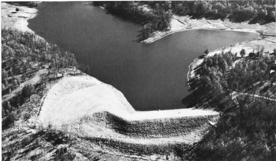
A floodwater-retarding structure on Six Mile Creek.
