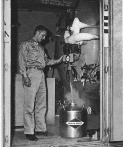
Recharging a technician's refrigerator with liquid nitrogen at a distribution point. The small refrigerator holds about 500 ampules of semen and enough liquid nitrogen for 2 weeks' storage. Frozen semen permits more efficient utilization of semen.
