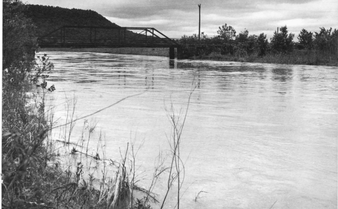
After channel improvements, Six Mile Creek flows at full capacity after a 6-inch rain.
