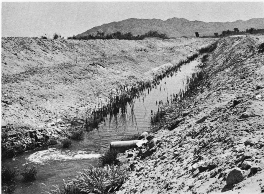
The tile outlet into a drainage ditch.
