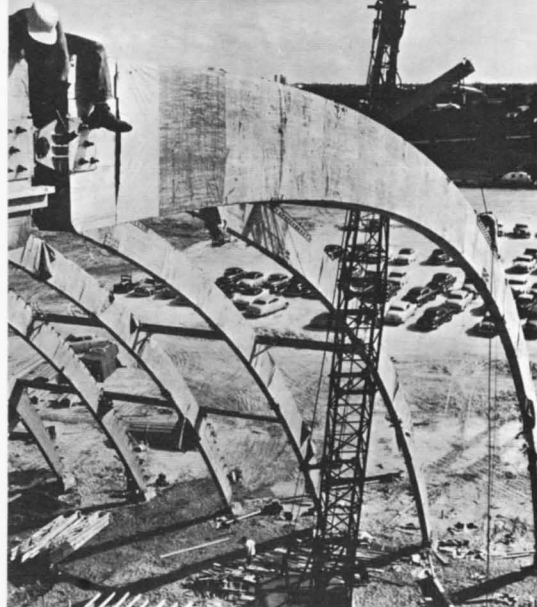
Improved gluing technology enabled engineers to extend the use of wood as an engineering material, like these huge laminated members.
