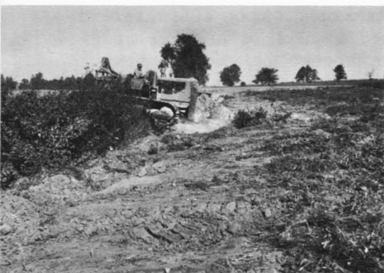
The gully was filled, and a waterway was developed.
