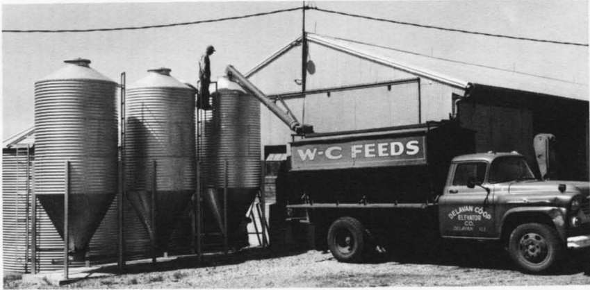
Purchased feed ingredients are delivered and stored in bulk. Automatically controlled auger conveyors deliver the ingredients to the grinding mill.
