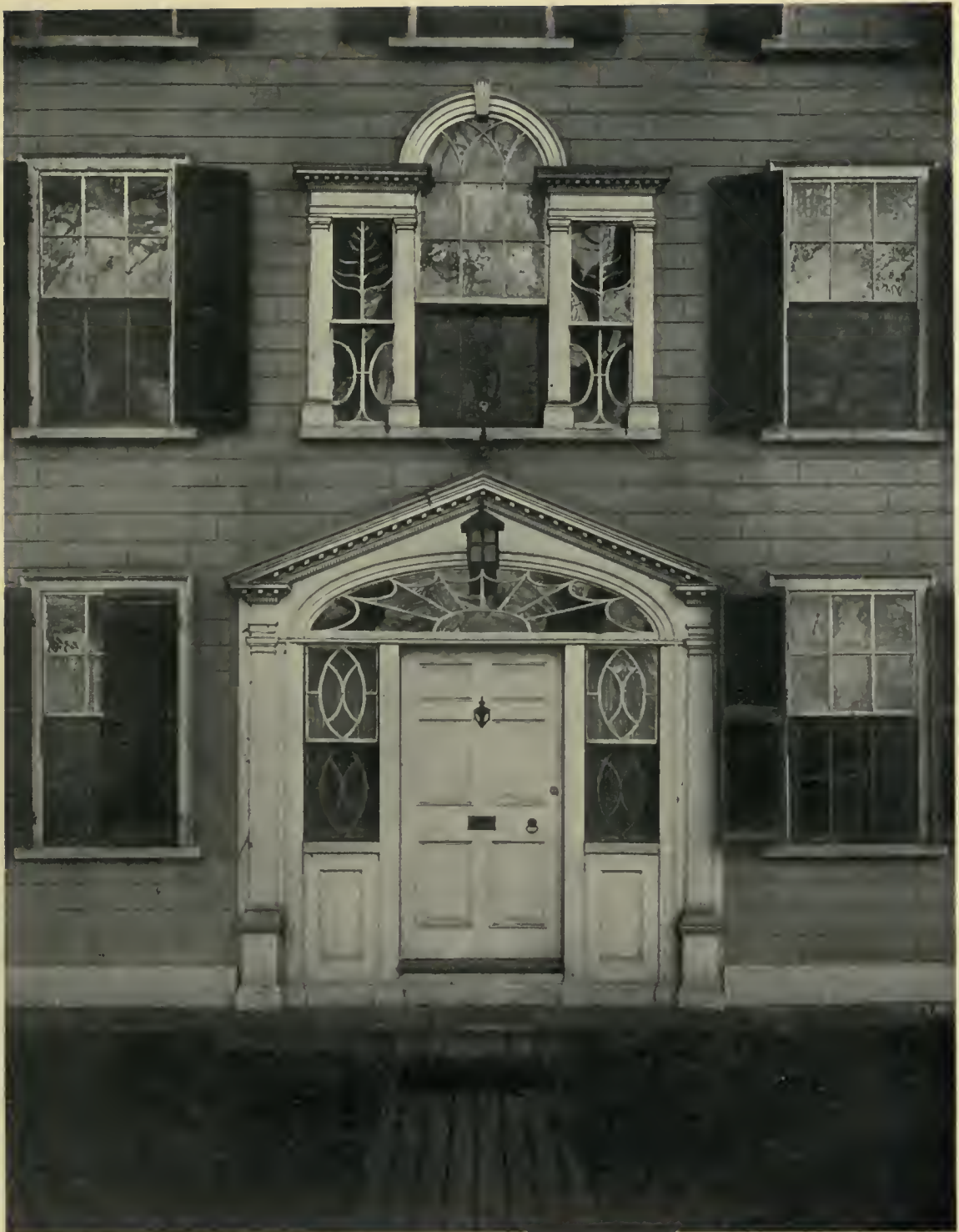
THE COLONEL LOAMMI BALDWIN HOUSE, WOBURN, MASSACHUSETTS. Detail of Entrance.
