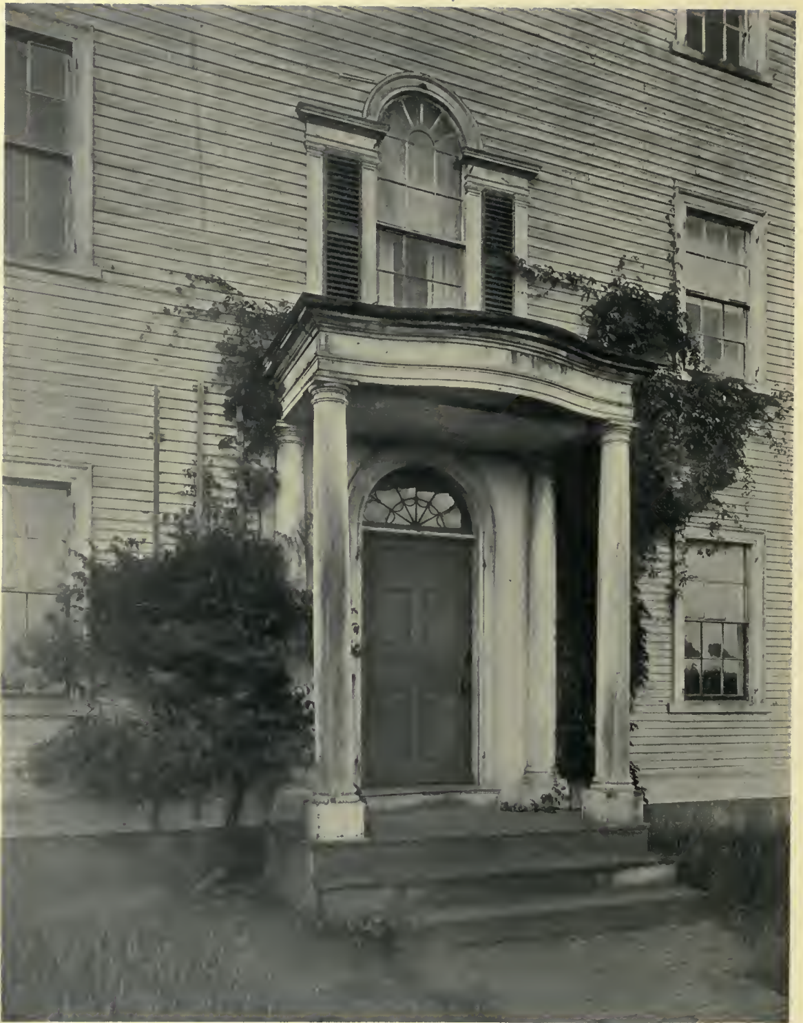
THE CROWINGSHIELD HOUSE AT DANVERSPORT, MASSACHUSETTS. (1798-1803.) Detail of Entrance.
