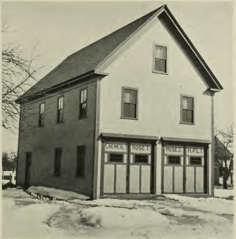
FIRE DEPARTMENT BUILDING, WEST ACTON Built in 1903
