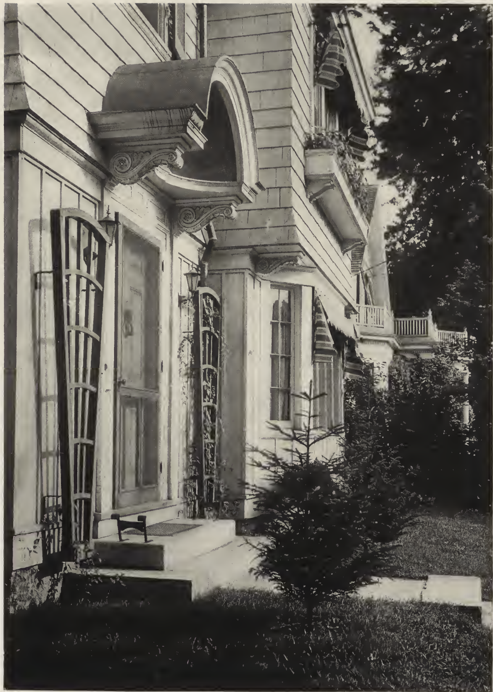
RESIDENCE OF DR. EDMUND F. CURRY, FALL RIVER, MASS. PARKER MORSE HOOPER, ARCHITECT.
