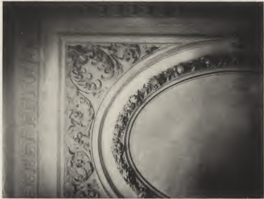
STAIRCASE CEILING—THE PYNES.
