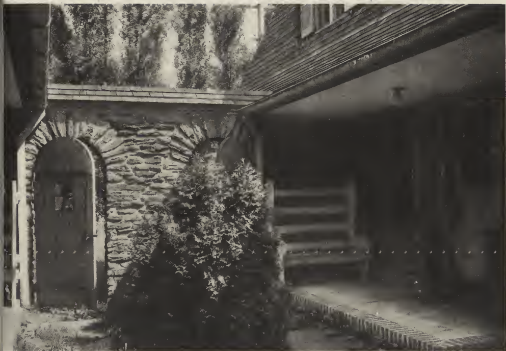
ENTRANCE COURT—PAIR OF SMALL HOUSES NEAR HAVERFORD, PA. Wilson Eyre & McIlvaine, Architects.
