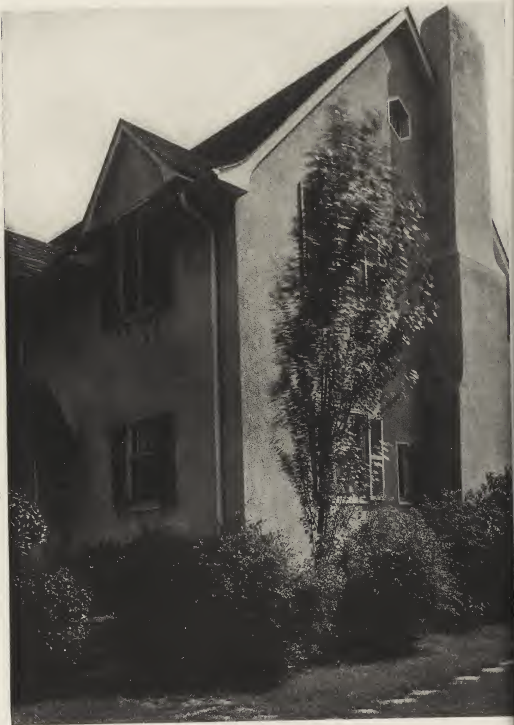
DETAIL OF FRONT—RESIDENCE AT HARTSDALE, N. Y. FRANK ARNOLD COLBY, ARCHITECT.
