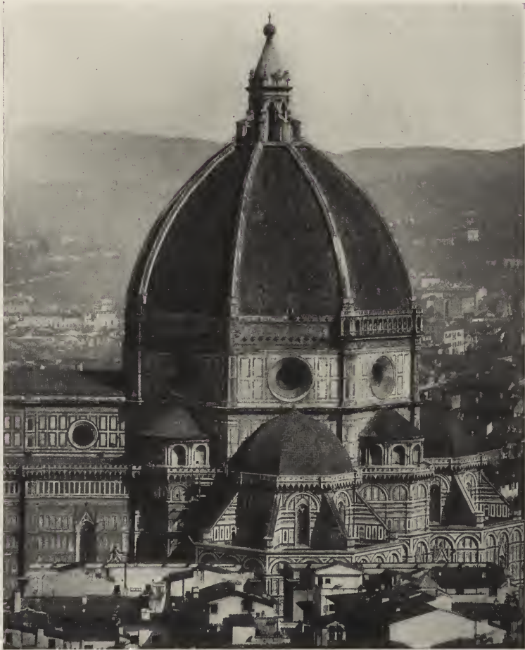
DOME OF CATHEDRAL OF FLORENCE. DESIGN EXPRESSES STRUCTURAL SYSTEM; INVISIBLE STRAINS RESISTED BY CONCEALED BELTS.
