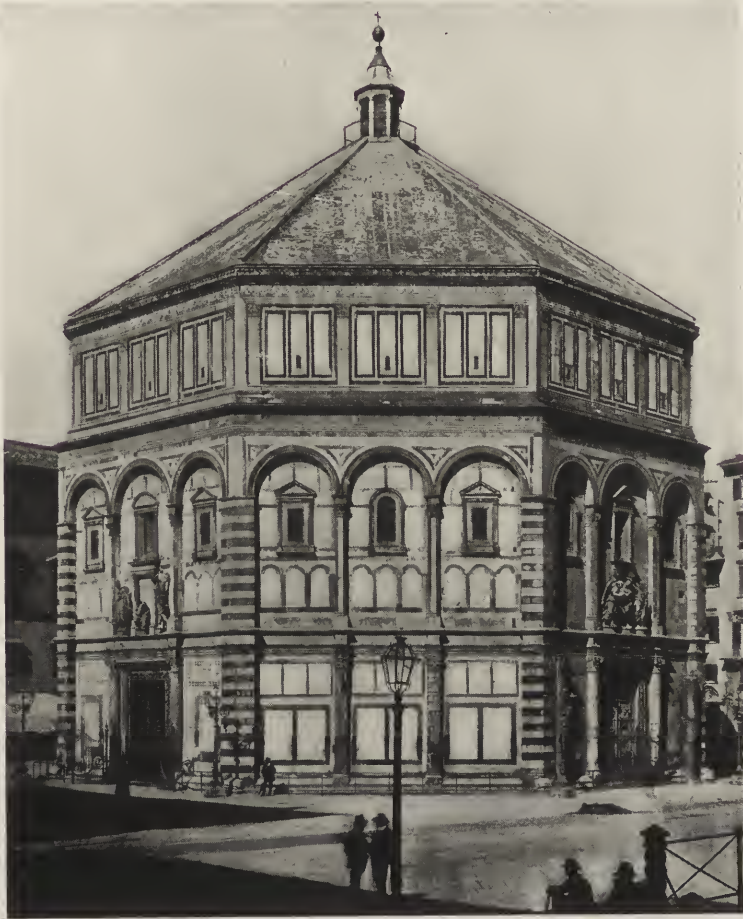
BAPTISTERY OF FLORENCE. DOME CONCEALED BY WALL OF DRUM CARRIED UP TO SUPPORT PYRAMIDAL ROOF.
