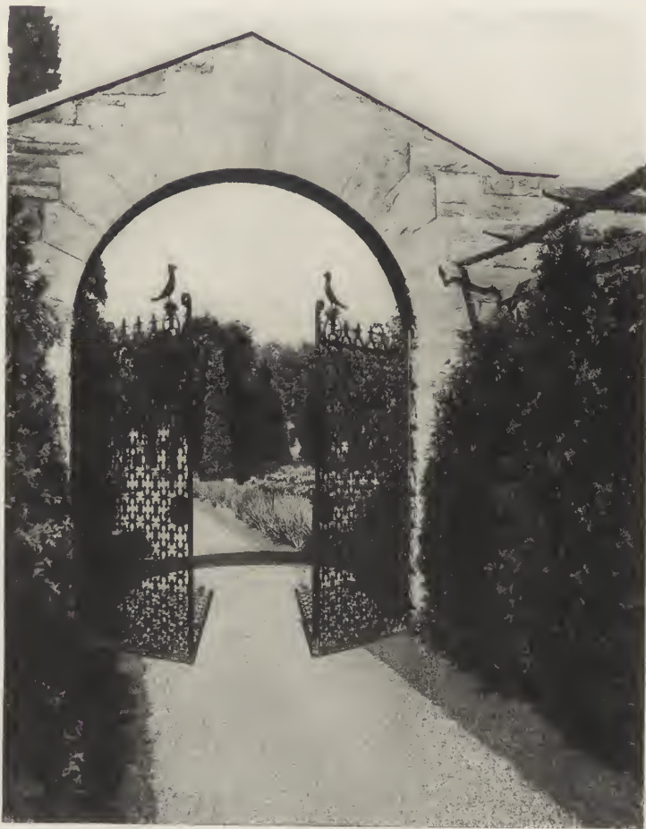
BLUE JAY GATE, OR THE VEHICLE ENTRANCE TO THE WHITE GARDEN. MASONRY OF NATIVE PATTON SANDSTONE IN WARM LIGHT-BROWN TINTS.
