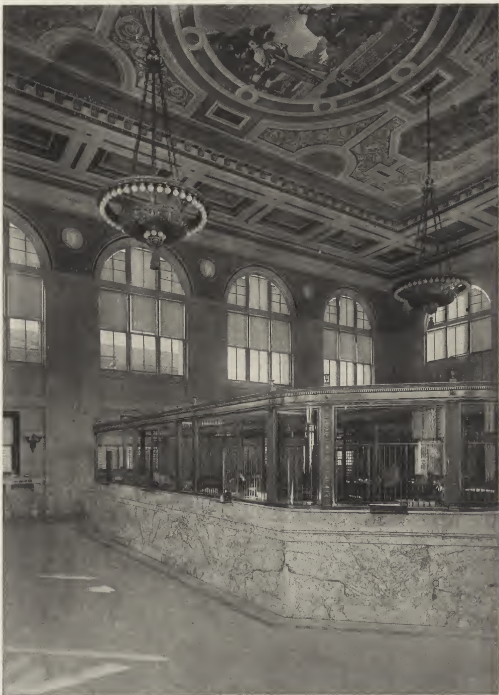
TITUSVILLE TRUST COMPANY'S BUILDING, TITUSVILLE, PA. ALFRED C. BOSSOM, ARCHITECT.
