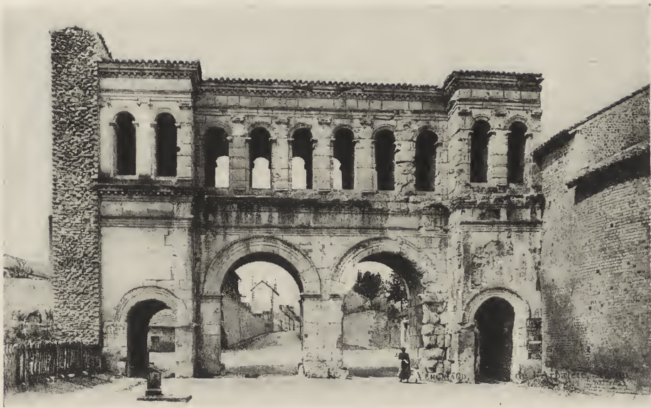
EXTERIOR—PORTE ST. ANDRÉ AT AUTUN.
