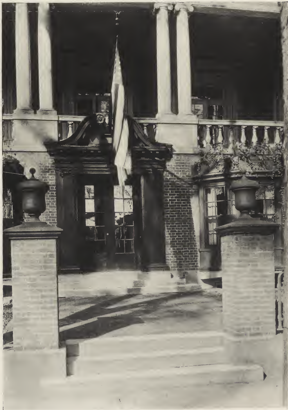
MAIN ENTRANCE—UNIVERSITY CLUB, SYRACUSE, N. Y. TAYLOR & BONTA, ARCHITECTS.
