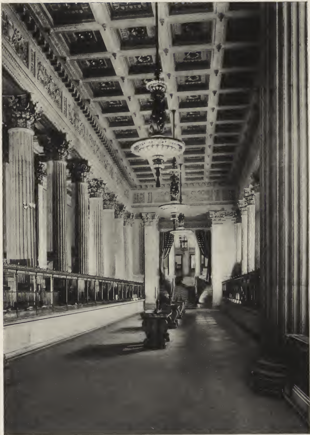
MAIN BANKING ROOM FROM VESTIBULE—GUARDIAN SAVINGS AND TRUST COMPANY'S BUILDING, CLEVELAND, OHIO. WALKER & WEEKS, ARCHITECTS.
