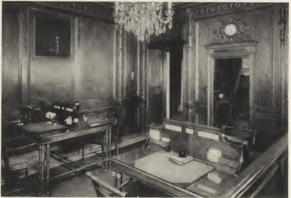
WOMEN'S ROOM—GUARDIAN SAVINGS AND TRUST COMPANY'S BUILDING, CLEVELAND, OHIO. Walker & Weeks, Architects.
