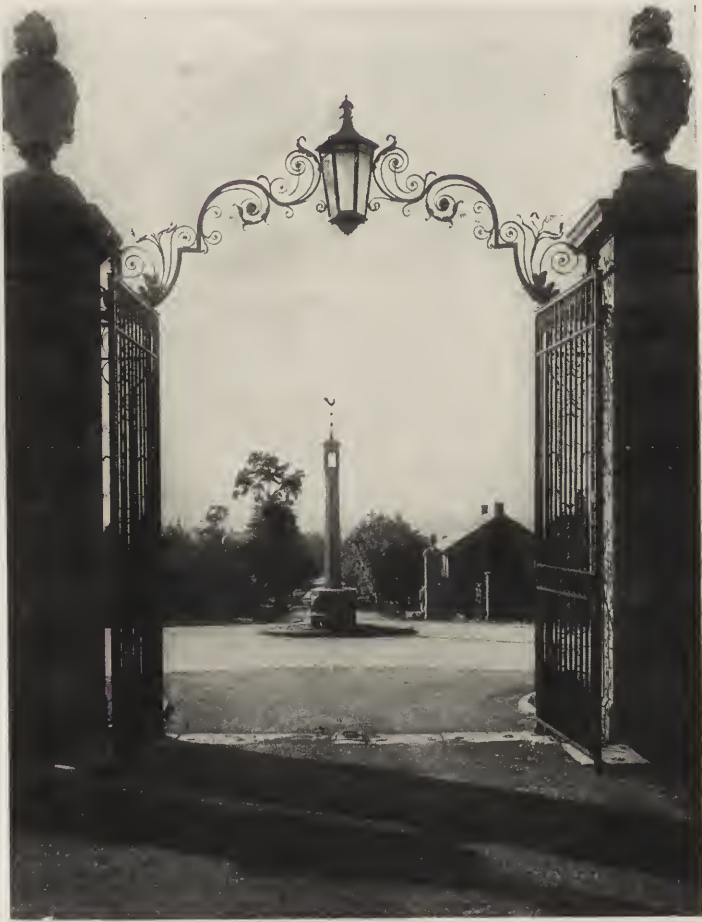
VIEW FROM MAIN ENTRANCE GATE ACROSS THE PIAZZA AT THE INTERSECTION OF THE STATE HIGHROAD WITH THE VILLAGE STREET.
