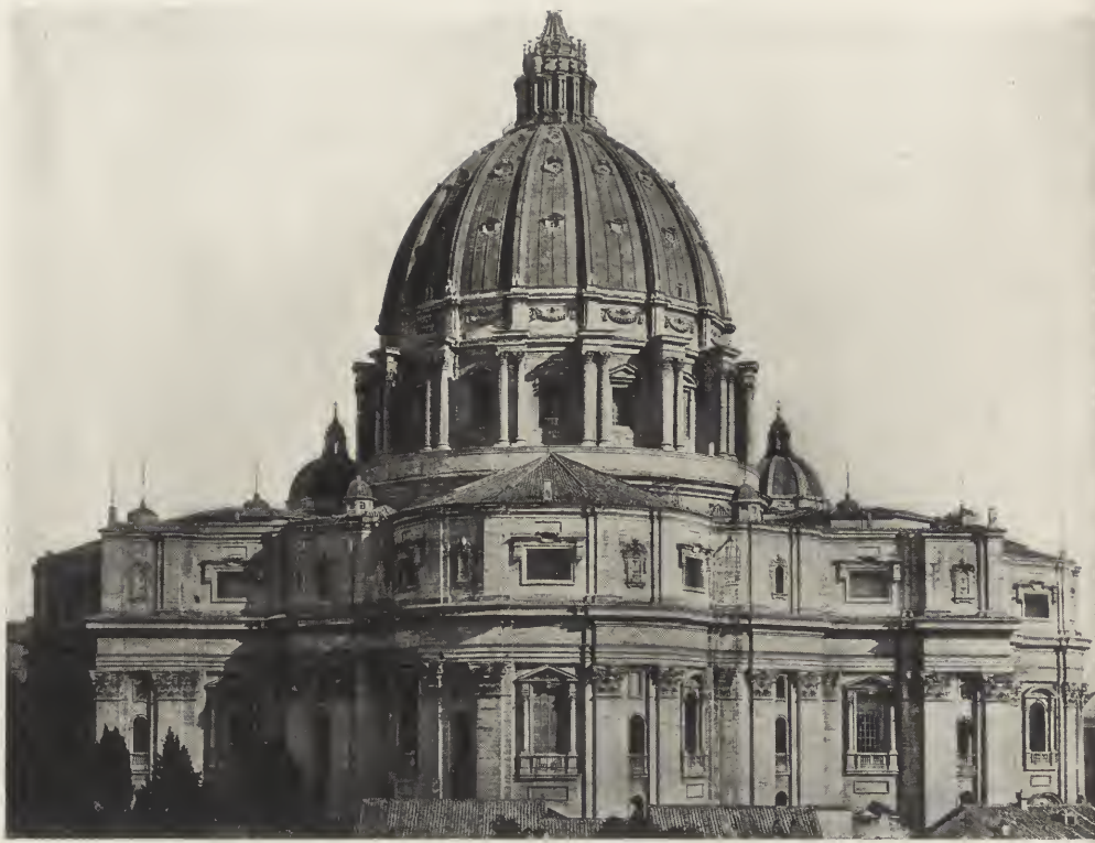
DRUM OF ST. PETER'S. BUTTRESSES OF DRUM PRODUCE SATISFACTORY EXPRESSION OF STABILITY.
