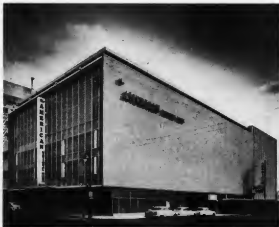
Fig. 5—The American National Bank building, Austin, Tex., showing all-brick and all-glass façades. Architects are the firm of Kuehne, Brooks, and Barr
