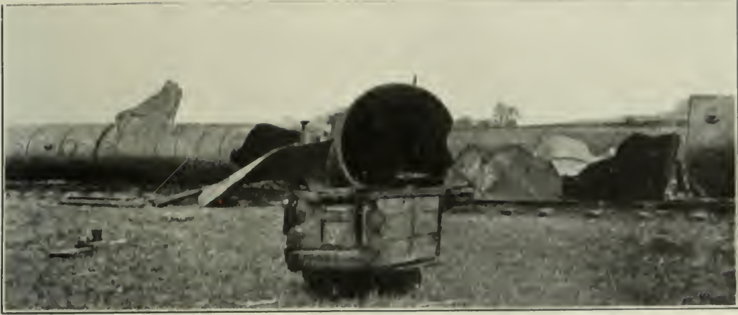
A. ALTOFTS EXPERIMENTAL GALLERY AFTER EXPLOSION OF DUST OCCUPYING 450 LINEAR FEET OF GALLERY, AUGUST 11, 1908.
