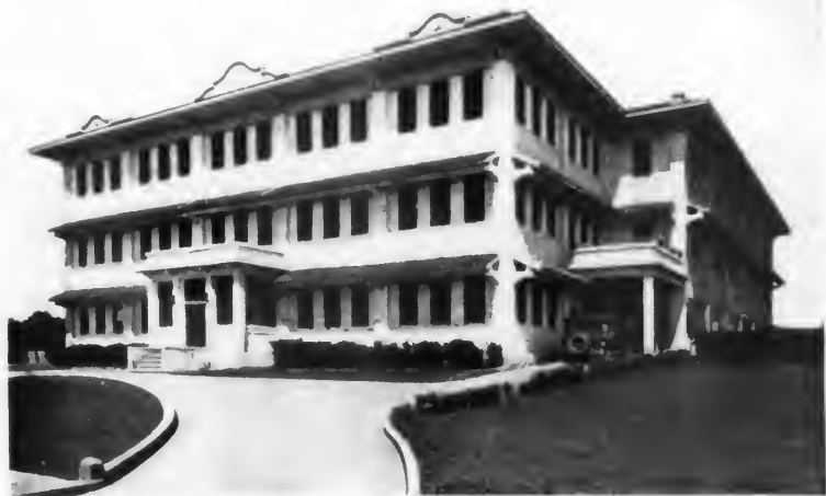
INTERNATIONAL HOSPITAL, CIUDAD TRUJILLO, DOMINICAN REPUBLIC One of the new institutions showing the development of hospital-mindedness in Latin America.
