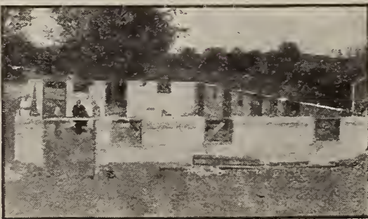
Foundation for C. C. Lubke's barn, Middleton
