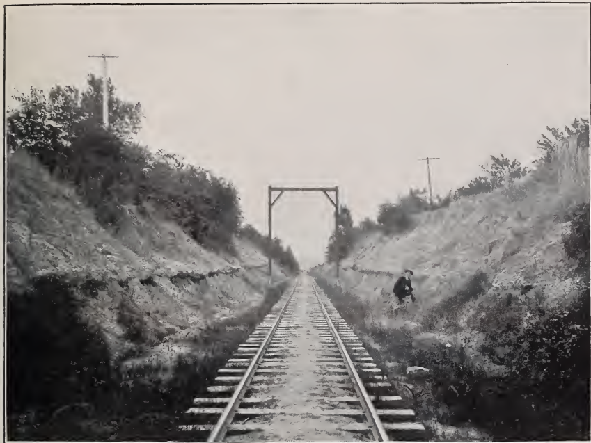
A. RAILROAD CUT AT LADONIA STATION.
