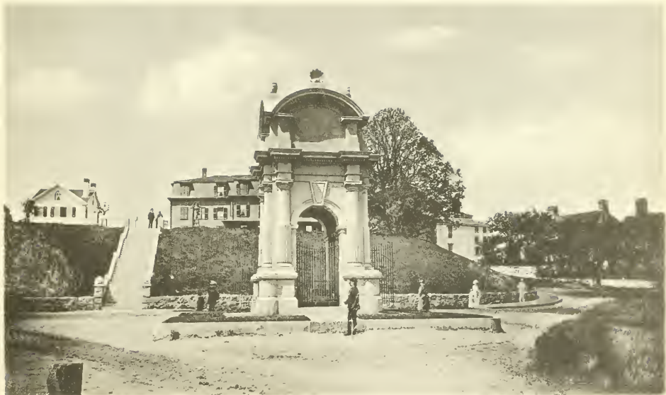
COLE'S HILL, THE FIRST BURIAL PLACE OF THE PILGRIMS. CANOPY OVER PLYMOUTH ROCK.
