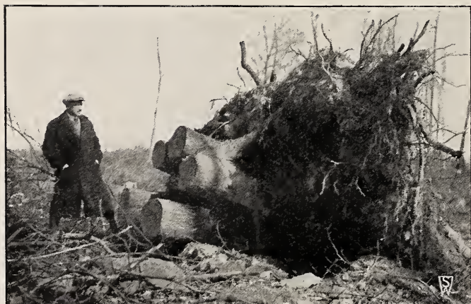
In construction work a deal of stump-pulling is often necessary; above shows the type of stump that the "K" hand stump-pulling outfit took care of at Canoebrook, N. J. Stump & Walter Co.'s seeds were used on this course.
