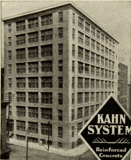
Mergenthaler Linotype Co. Bldg., Brooklyn, N. Y. Kahn System Reinforced Concrete.
