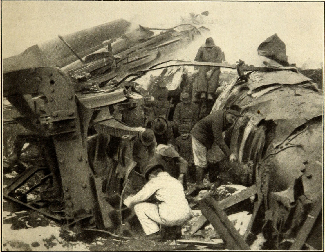
WRECK OF THE WHITE MOUNTAIN EXPRESS ON THE NEW YORK, NEW HAVEN, AND HARTFORD RAILROAD, AT GREENWICH, CONNECTICUT, IN 1908. SPREADING RAILS WERE THE CAUSE OF THIS ACCIDENT. ONE WOMAN WAS KILLED AND 25 PERSONS INJURED
