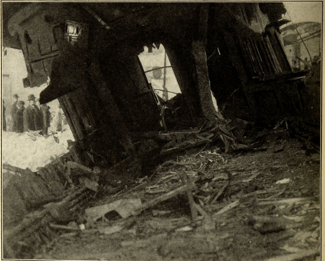
INSIDE OF A SLEEPING-CAR AFTER A WRECK ON THE NEW YORK CENTRAL RAILROAD
