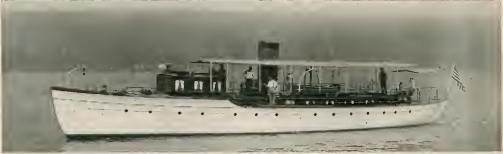
Drusilla is 83 feet long with a beam of 14 feet and a 4-foot draft.
