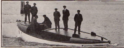
Running with Cabin Compartment Pumped Full of Water
