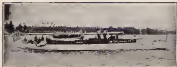
No. 3693.—90 ft. steam yacht. Suitable for ferry service. Speed 18-20 miles. Bargain.
