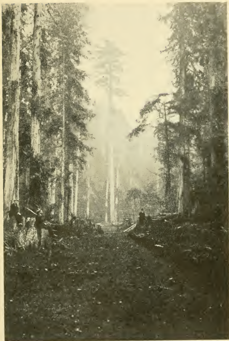
Sub-grade for motor truck logging road.
