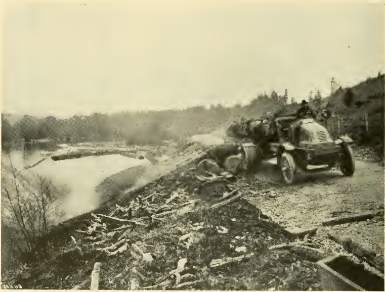
Unloading truck and trailer through the use of an incline, showing brow-skids and roll-way.
