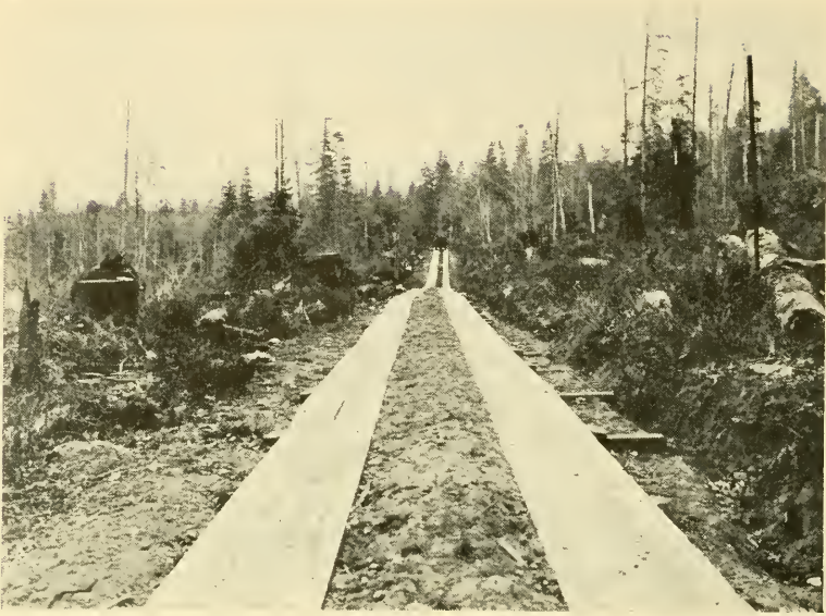
Fore-and-aft plank road with wedges on cross ties to facilitate the re-aligning of the planks.
