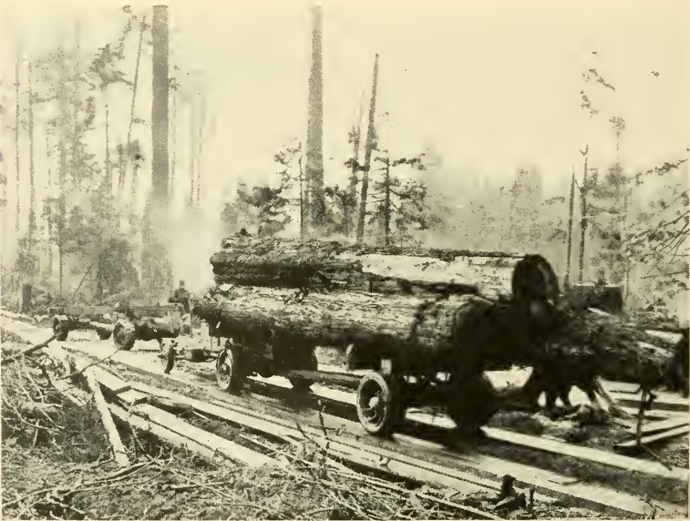
Turn-out on fore-and-aft plank road.
