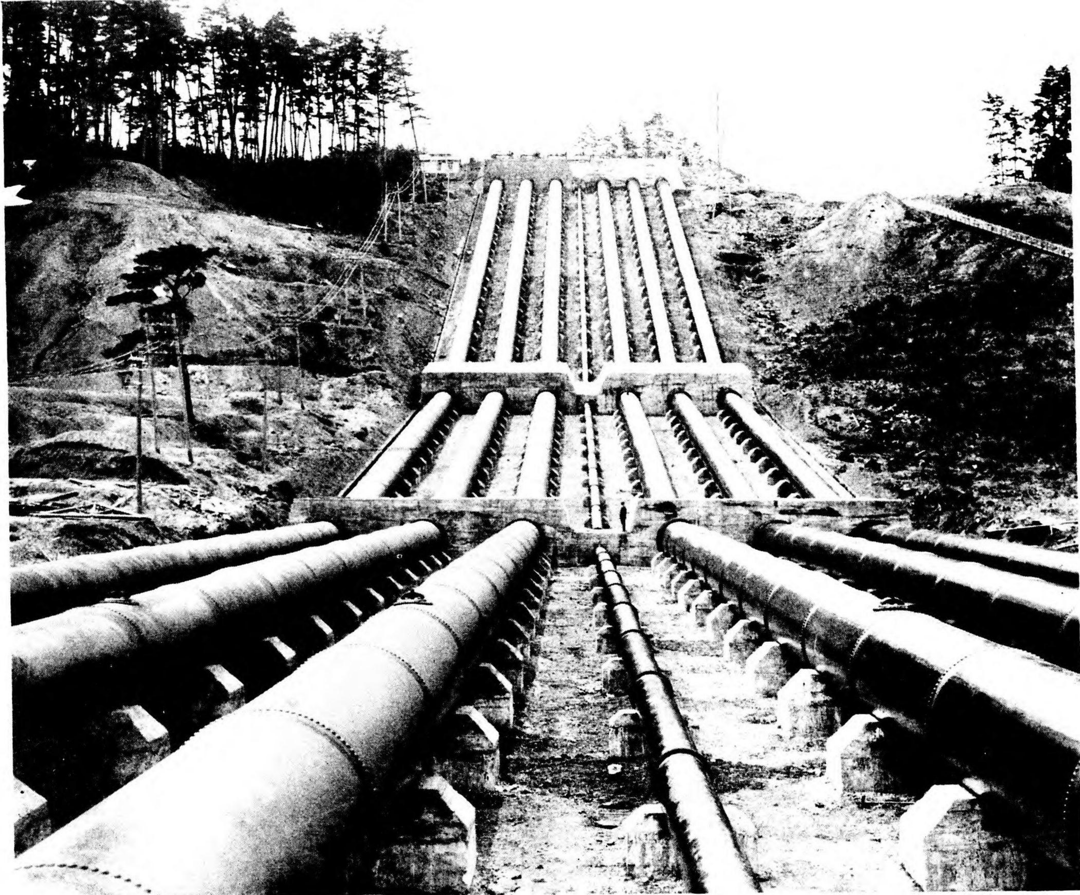
Fig. 27—Penstocks. Target No. 90.10-881. Those of more recent construction are welded at the joints instead of riveted. The small pipe line is for operation of pressure governors.
