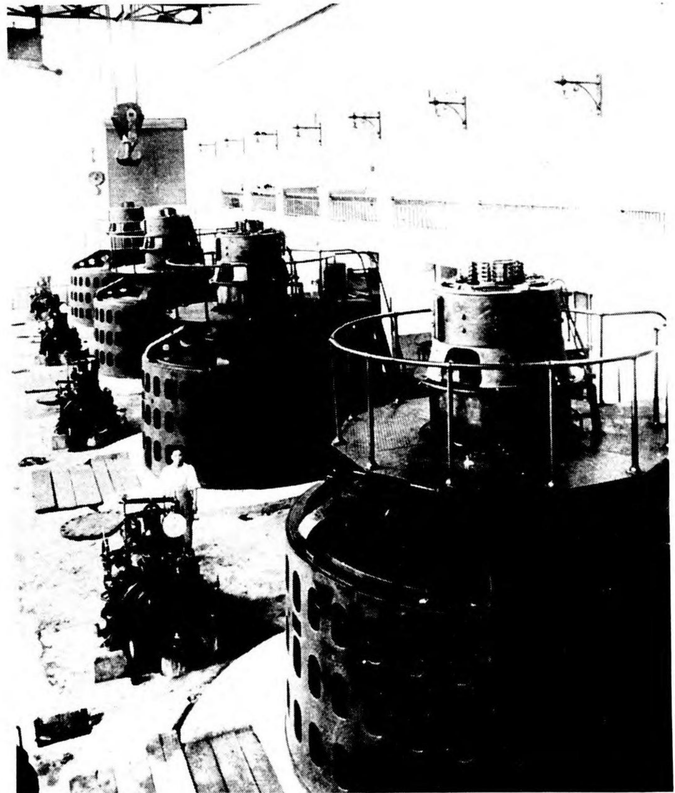
Fig. 24. Right: Target No. 90.20-1144 Vertical generators in the turbine room of the Seto Hydro Electric Station.
