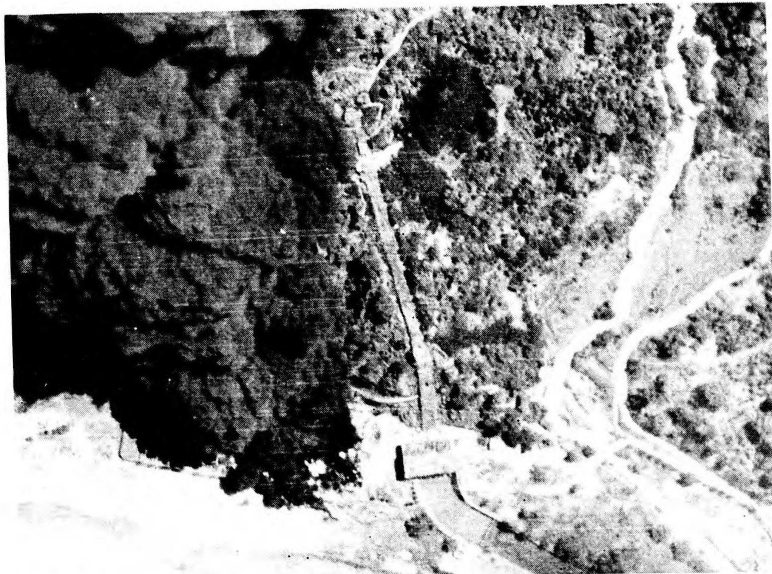
Fig. 31—Target No. 91.4-83 Jitsugetsutan Power Plant No. 2. An oil fire has engulfed the entire transformer yard and the lower section of a penstock has been ruptured.
