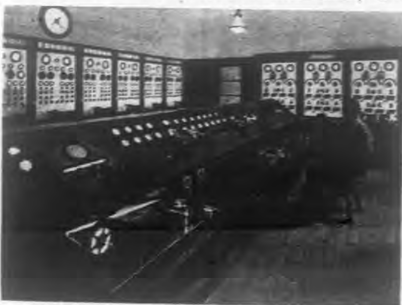
Telegraphs a few decades later: The control room of the central fire station of the city of Berlin, where, by a most elaborate telegraph installation of the Siemens System, the fire detection and reporting services of the metropolis are most efficiently concentrated
