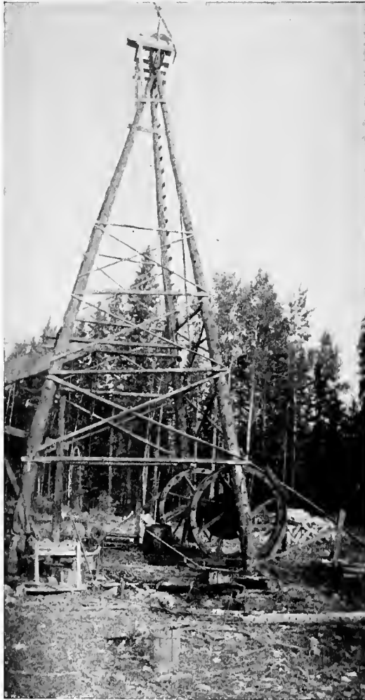
FIG 51. Pole rig used for drilling on the Athabasca River in northern Alberta, Canada.
