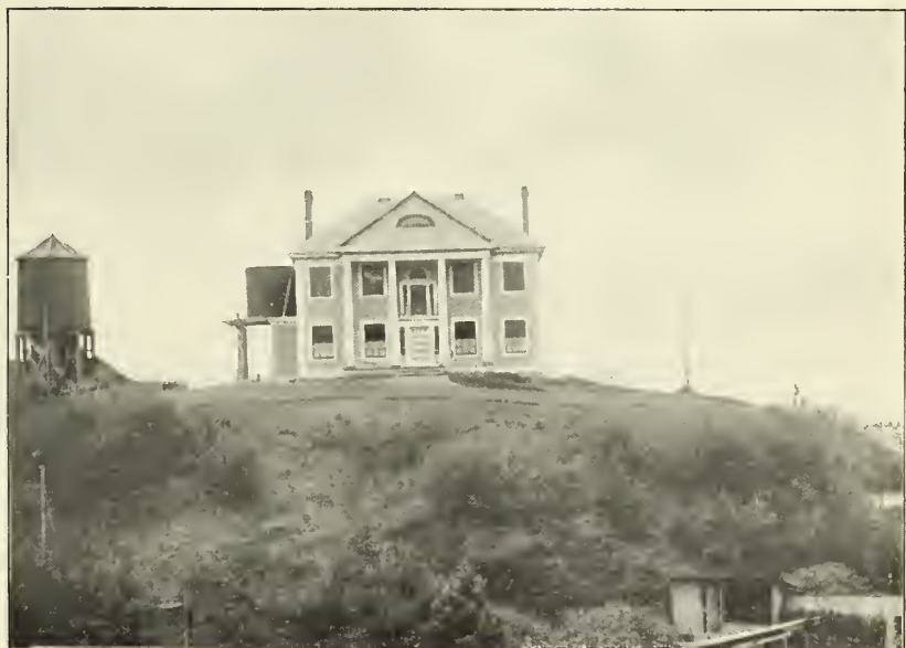
FIG. 2.—ALASKA STATIONS—STATION BUILDING, SITKA.
