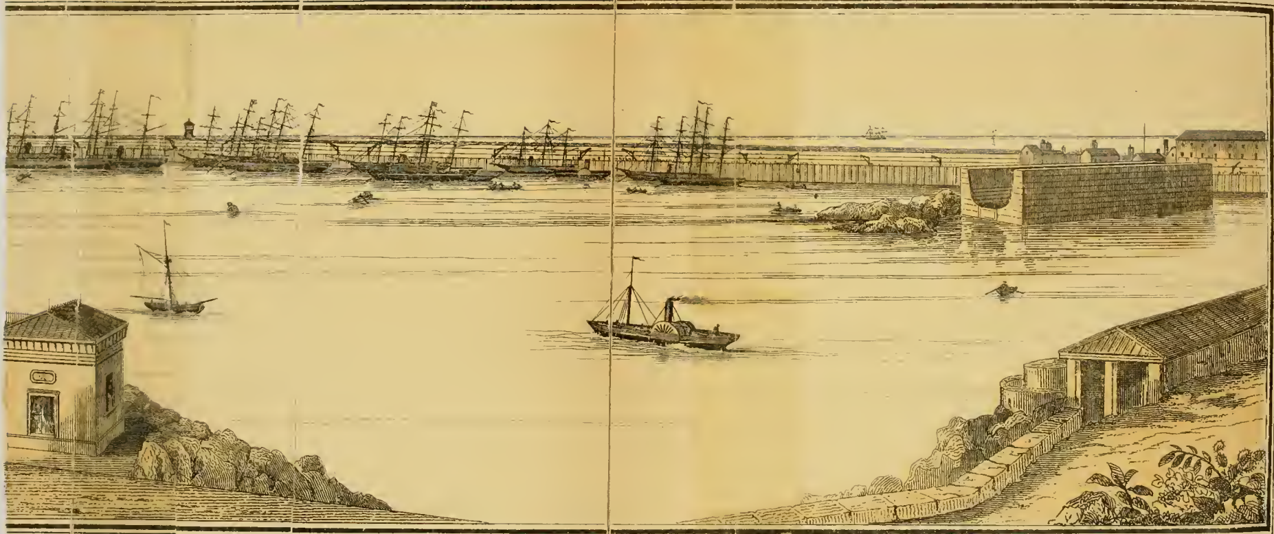
ER IN COURSE OF CONSTRUCTION AT PONTA DELGADA. (Taken from a Photograph).
