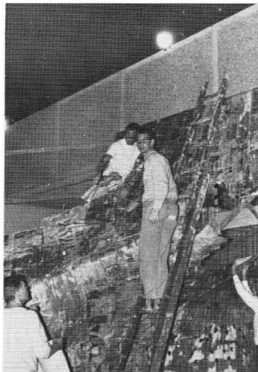
The wall goes higher.
