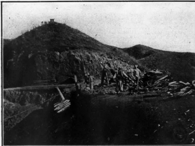
"TRIPPING" LOAD OF CORDWOOD BY CABLE
