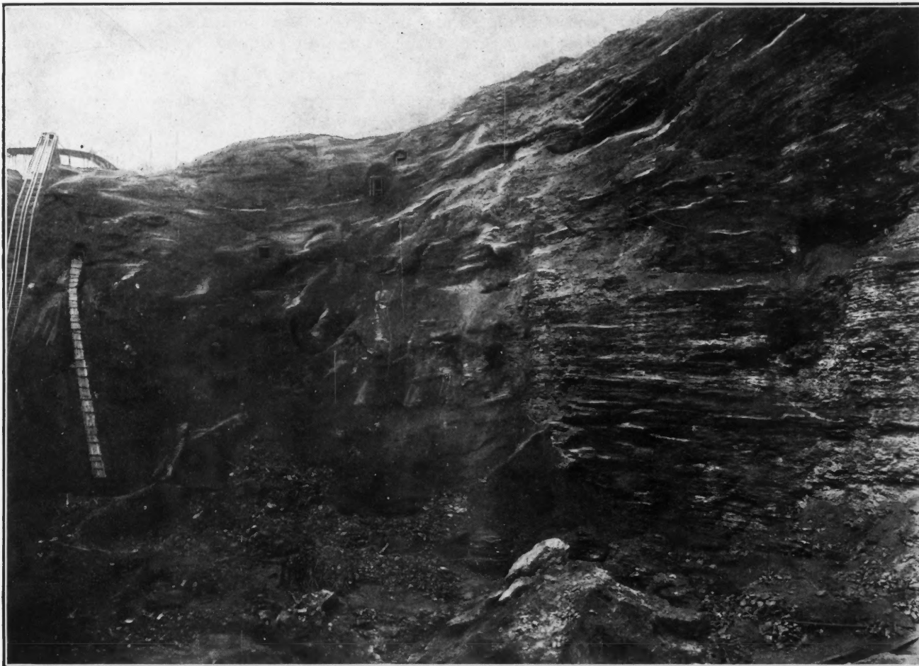
FIG. 8. SHARP ROCK-WALL OF A DEEP TROUGH OREBODY ON THE EAST CENTRAL PART OF THE RANGE Note face of wall. Left half of picture shows ore
