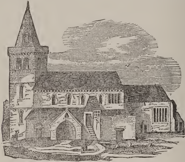
Crail Church (before the restoration).
