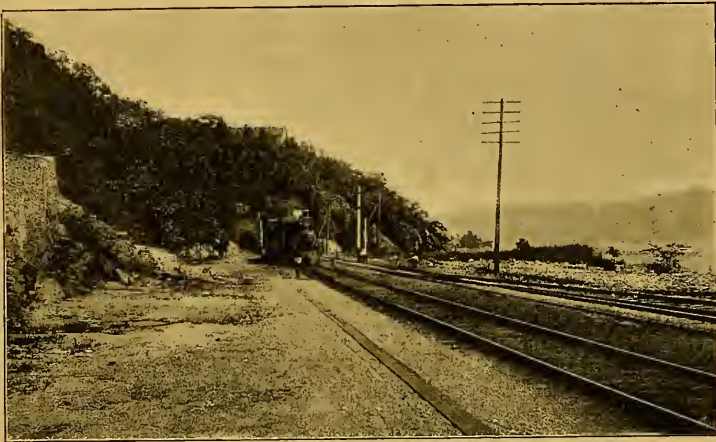
FIG. 2. TUNNEL UNDER WEST POINT.
