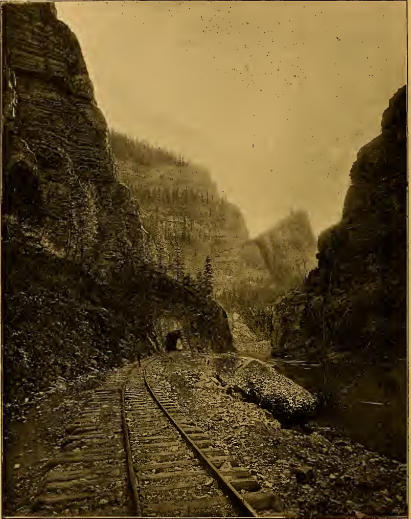
FIG. 46. TUNNEL ON THE GRAND RIVER CANON.
