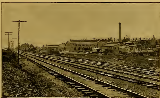
FIG. 97. NORTHERN PACIFIC RAILWAY SHOPS, TACOMA.
