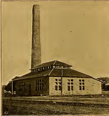
FIG. 68. POWER HOUSE, LELAND STANFORD UNIVERSITY.
