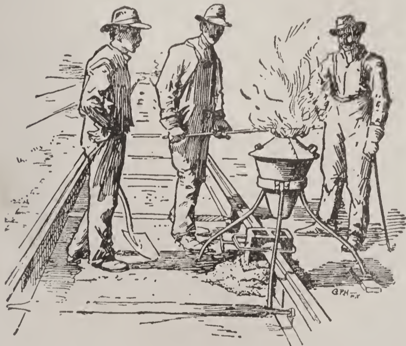
JOINING RAIL ENDS BY THE USE OF "THERMIT."
