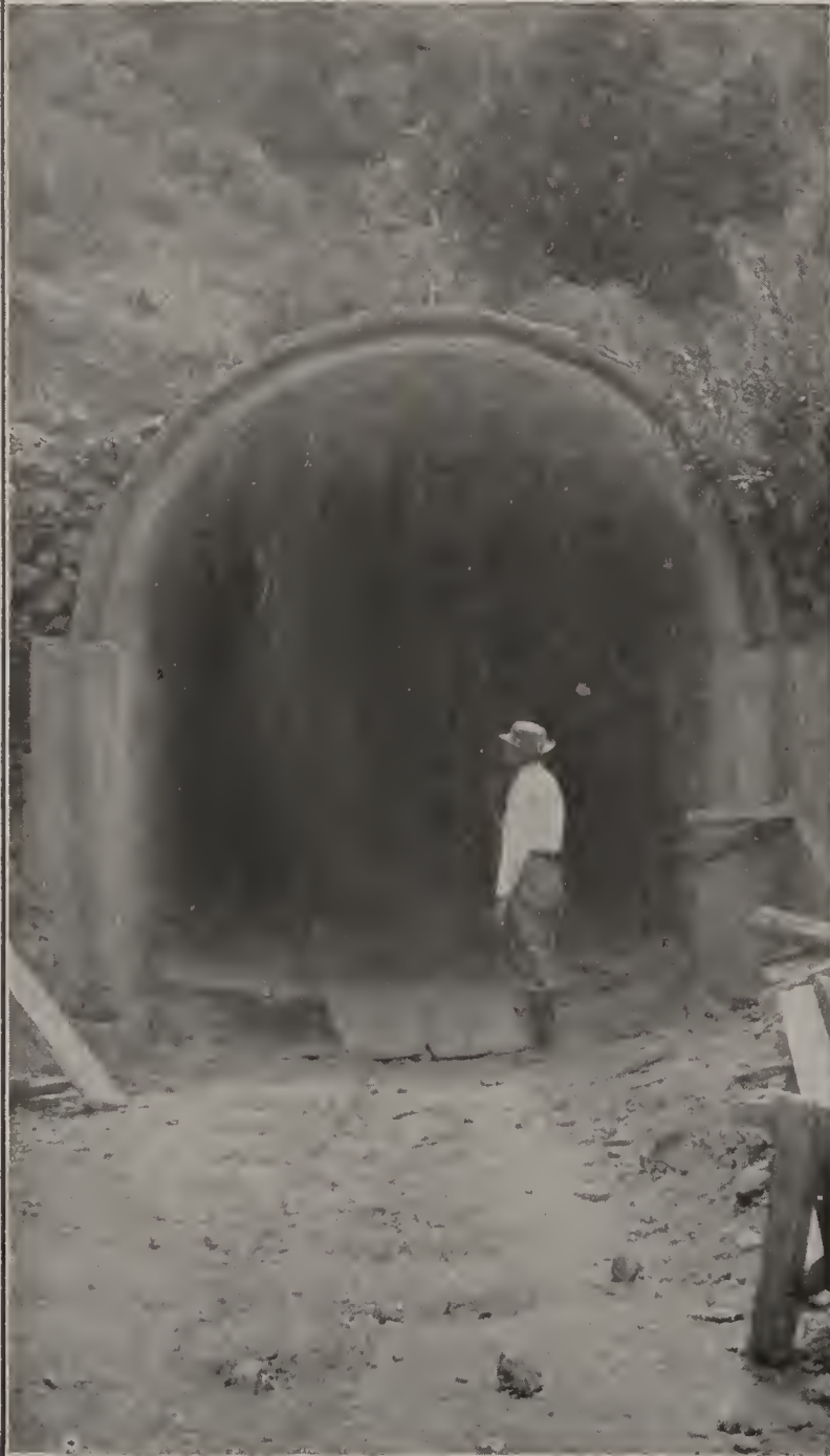
One of the aqueduct tunnels in the Langas division.
