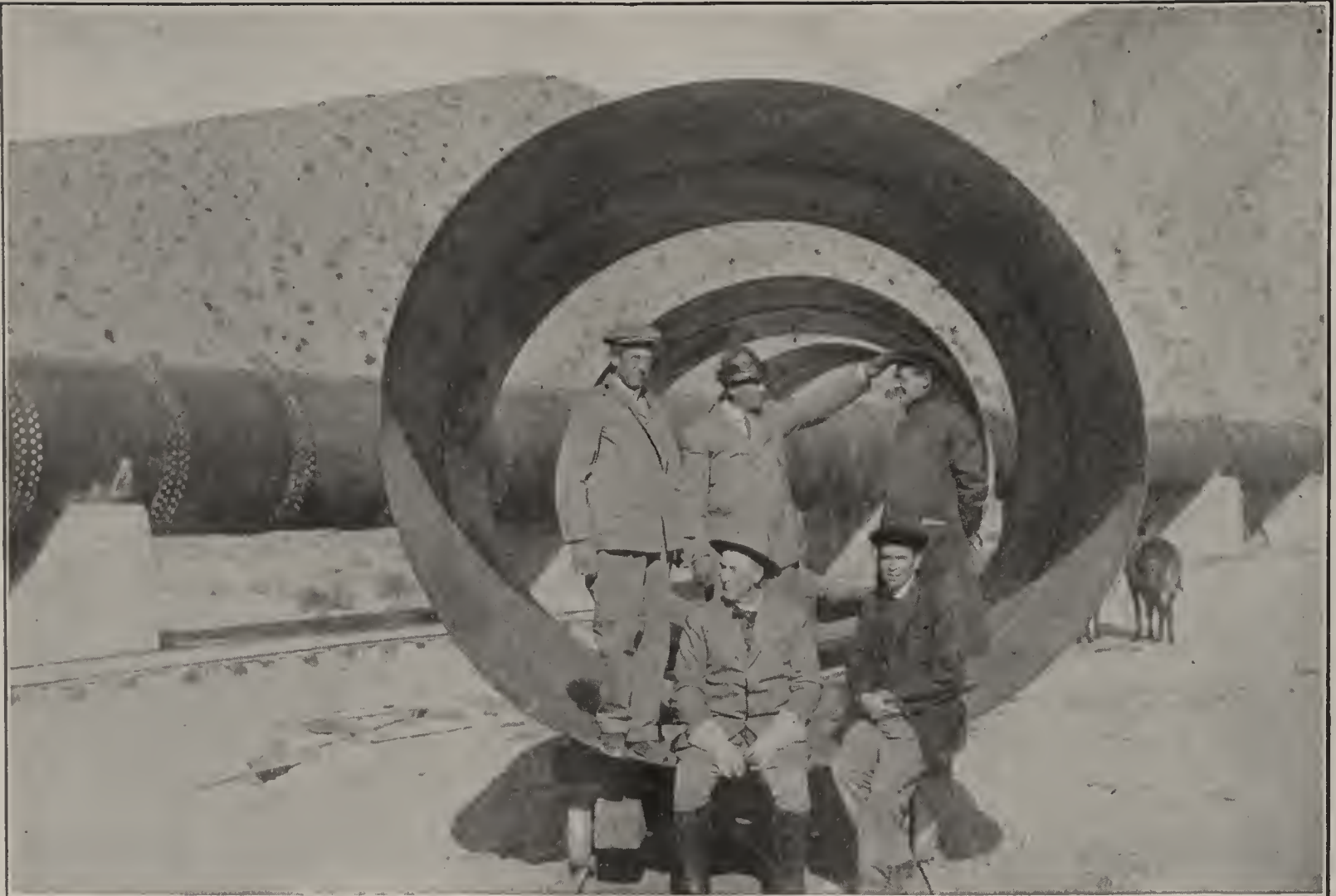
A section of the Antelope siphon showing steel pipe ten feet in diameter.
