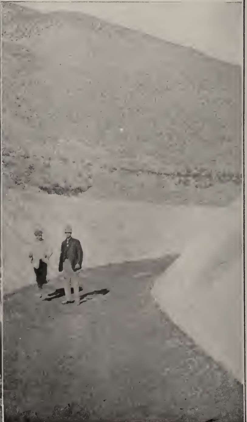
Open concrete lined ditch above Haiwee Reservoir.
