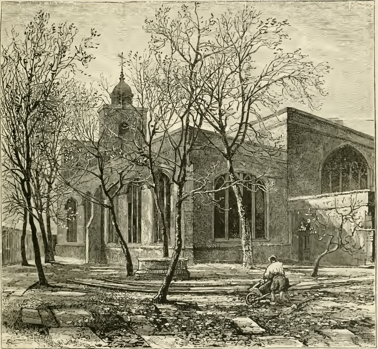
ALL HALLOWS BARKING, GREAT TOWER STREET.
