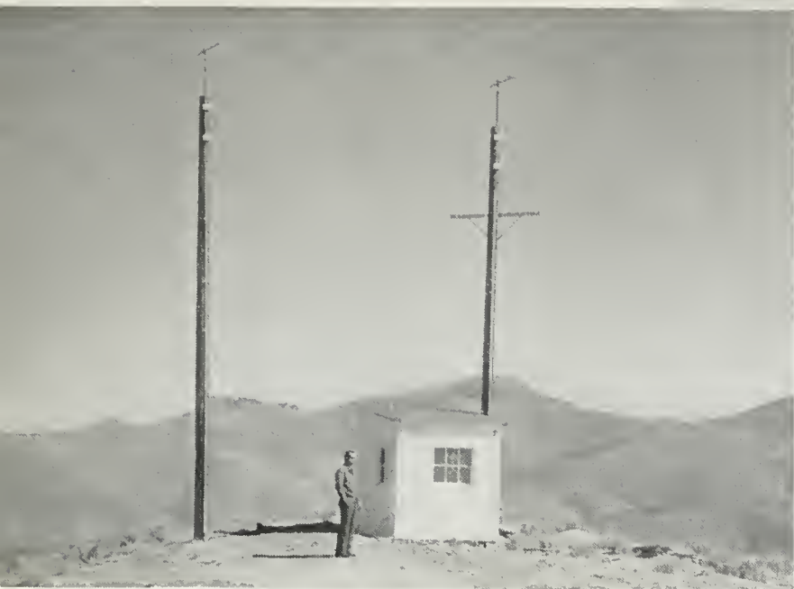
This radio relay station for rural service handles telephone calls to and from an isolated industrial enterprise in Nevada. The station at the right, on Mt. Blyn, Wash., speeds telephone calls across the waters to Victoria, B. C., replacing submarine cables
