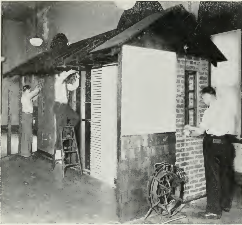
Typical residential construction, both exterior and interior, is simulated for these budding installers to practice on
