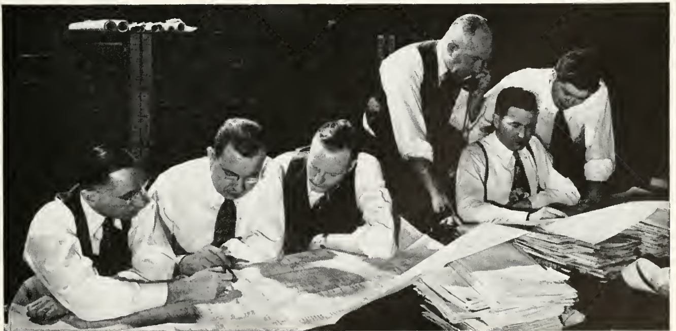
When this picture was taken, these engineers at the Kearny Works of the Western Electric Company were planning the emergency replacement of switchboards serving more than 10,000 telephones, which had been destroyed by fire
