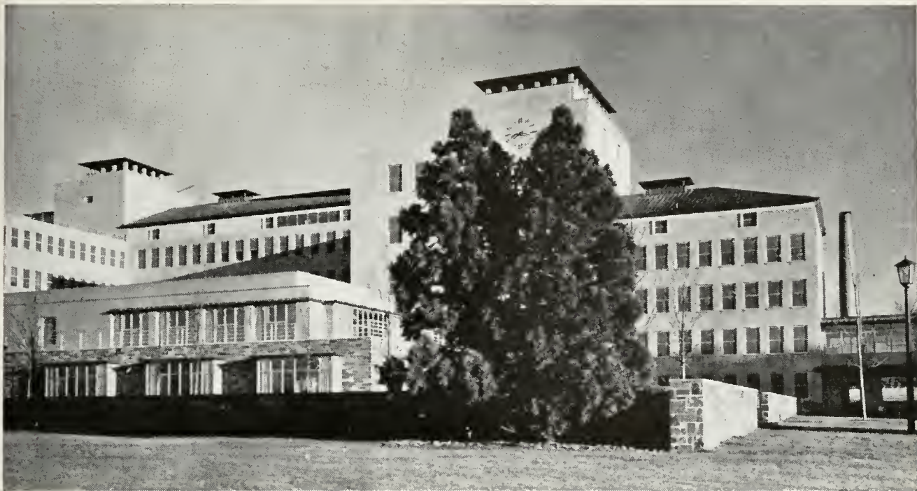
Part of the Murray Hill, N. J., installation of the Bell Telephone Laboratories
