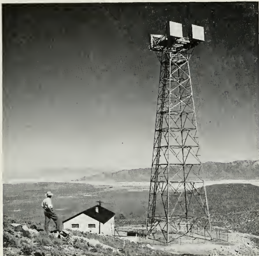
Six channels are now in operation on the transcontinental radio relay route, transmitting television and several hundred telephone conversations. This tower is at Cedar Mountain, Utah
