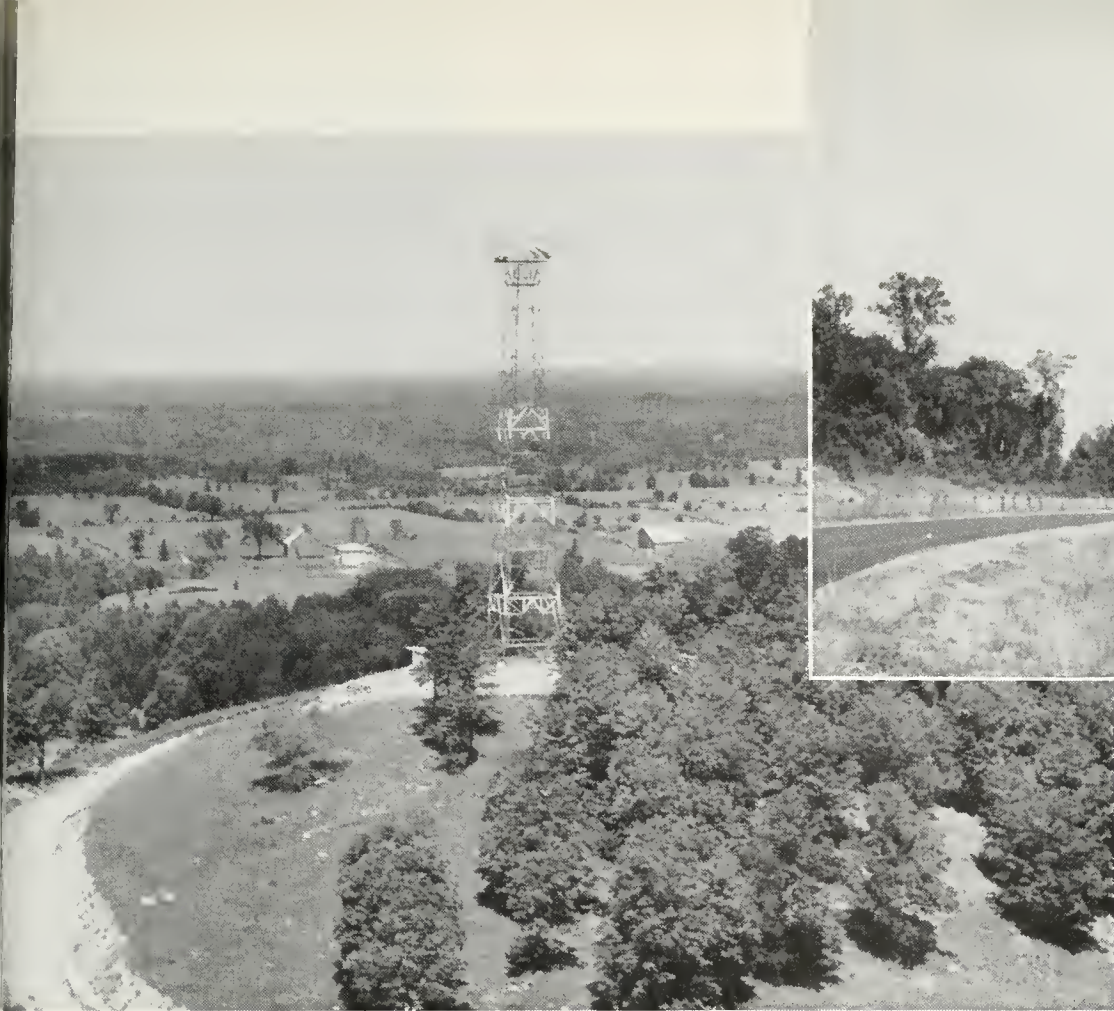
Access to radio relay equipment at the towers is essential. The road seen above was built for that purpose in Ontario, Canada, while it was possible to locate the tower at the right beside a highway in Georgia
