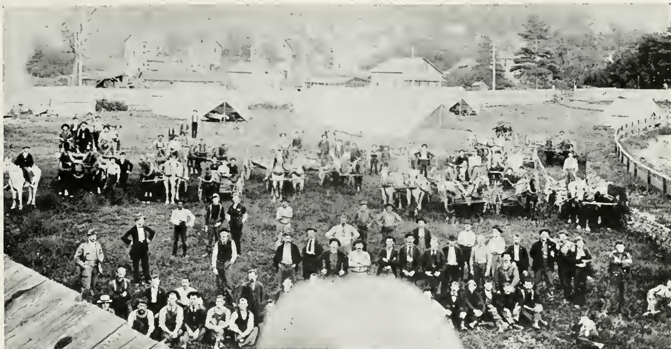
The men and equipment under Foreman J. O. Murphy line up for a photographer (atop a building in the fair grounds at Ridgeway, Pa.) to show what the well-set-up construction gang looked like in 1896
