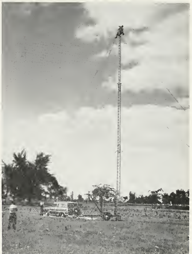
Bell System engineers use a balloon and a portable tower to select sites for microwave radio telephone stations for a private-line radio telephone system being installed for a major power company
