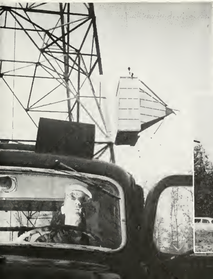
Lens antennas are big, heavy, and difficult to handle. The truck driver is watching signals in the mirror in his truck cab as he winches one aloft. That one is in New Jersey; the array of four is in Tennessee
