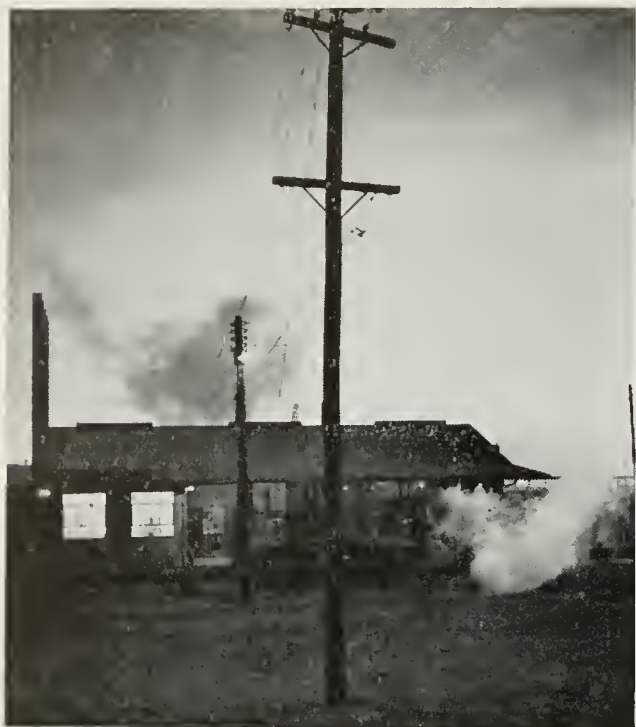
Pipe line pumping stations, impressive and often remote installations, receive operating instructions from their dispatchers over specially designed telephone circuits
