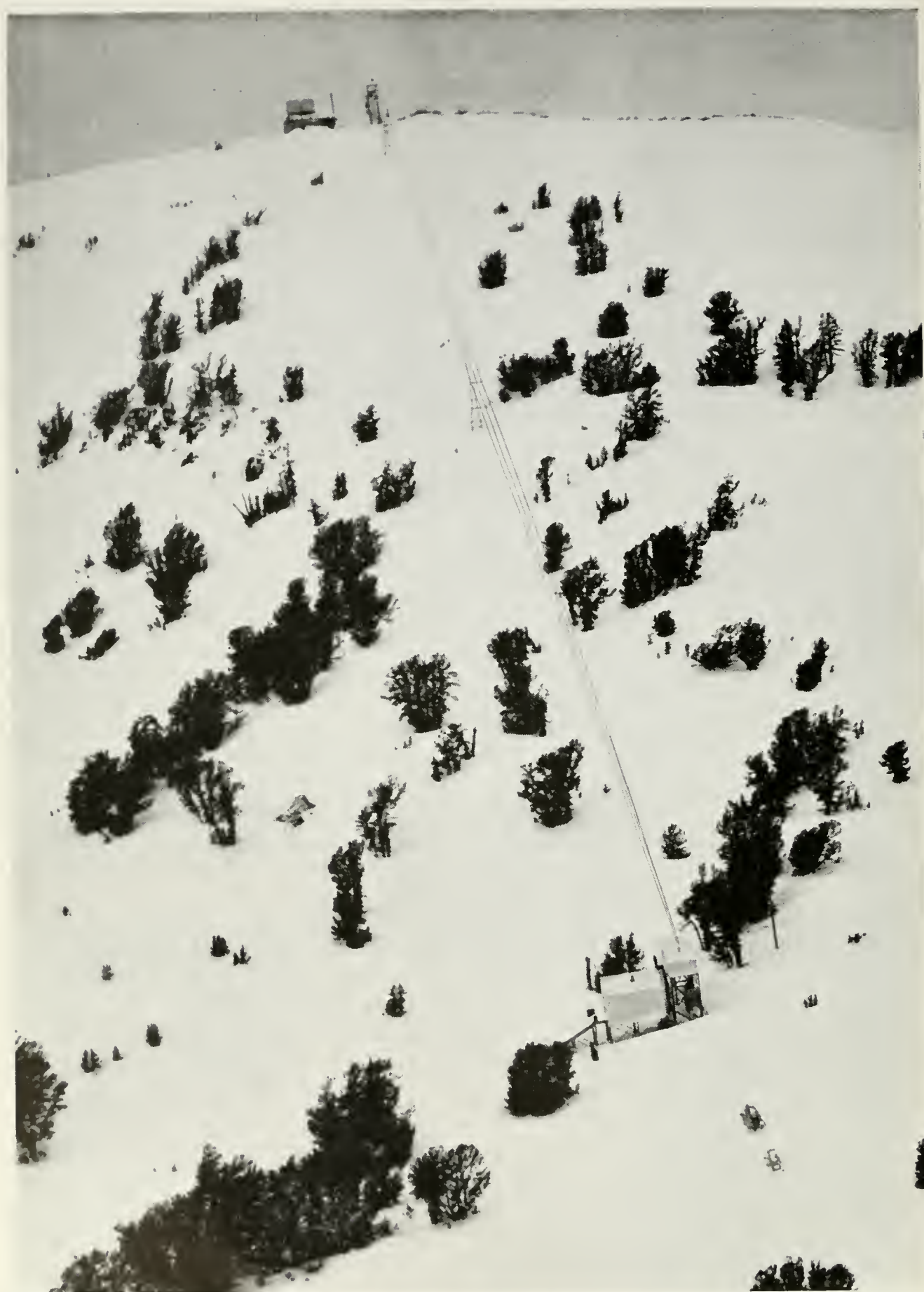
Except during the short summer season, the last quarter mile of the approach to the Mt. Rose radio relay station is by aerial tramway. Note the "sno-cats" at the lower right approaching the ramp and shelter over 10 feet of snow. See page 87
