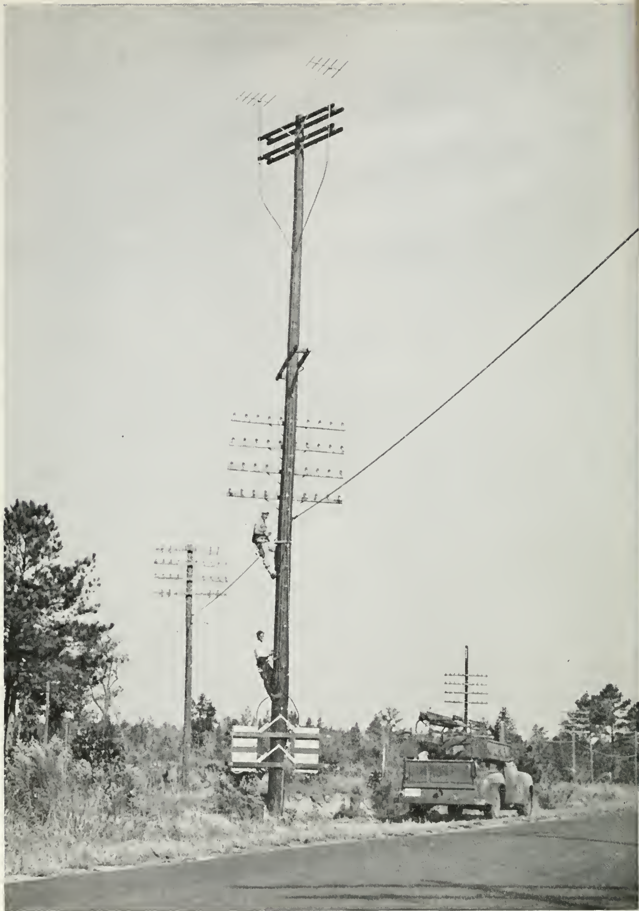
Versatile communications bearer: This single pole near Wilmington, North Carolina, supports open wire circuits, both voice frequency and carrier; cable circuits; and a radiotelephone transmitting installation. The radio provides telephone connection with Shallotte, more than 30 miles distant. See the article beginning on page 149
