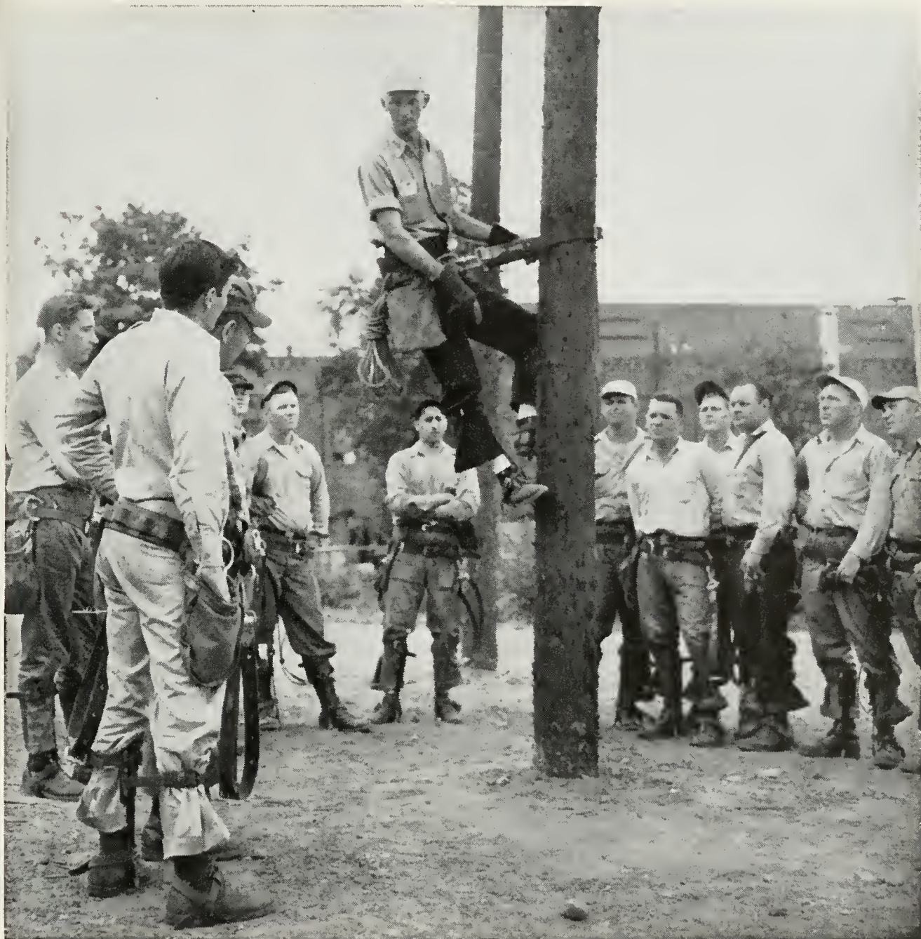
An instructor demonstrates the techniques of pole climbing. Soon each pupil will be proving his proficiency under the expert's watchful eye
