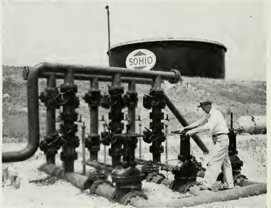
He proceeds outside and makes the necessary adjustment to the valve
