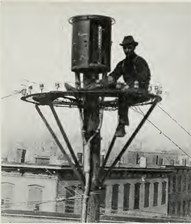
An example of terminal pole construction in the 1890s
