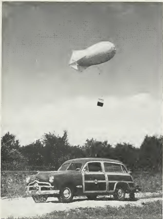
Bell System engineers use a balloon and a portable tower to select sites for microwave radio telephone stations for a private-line radio telephone system being installed for a major power company
