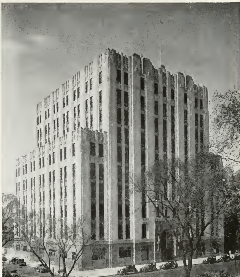
Bell System buildings—such as this of the Ohio Bell Telephone Company in Dayton—are architecturally appropriate to their surroundings, and in their substantial character and careful planning reflect the stability of the business and its regard for customers and employees
