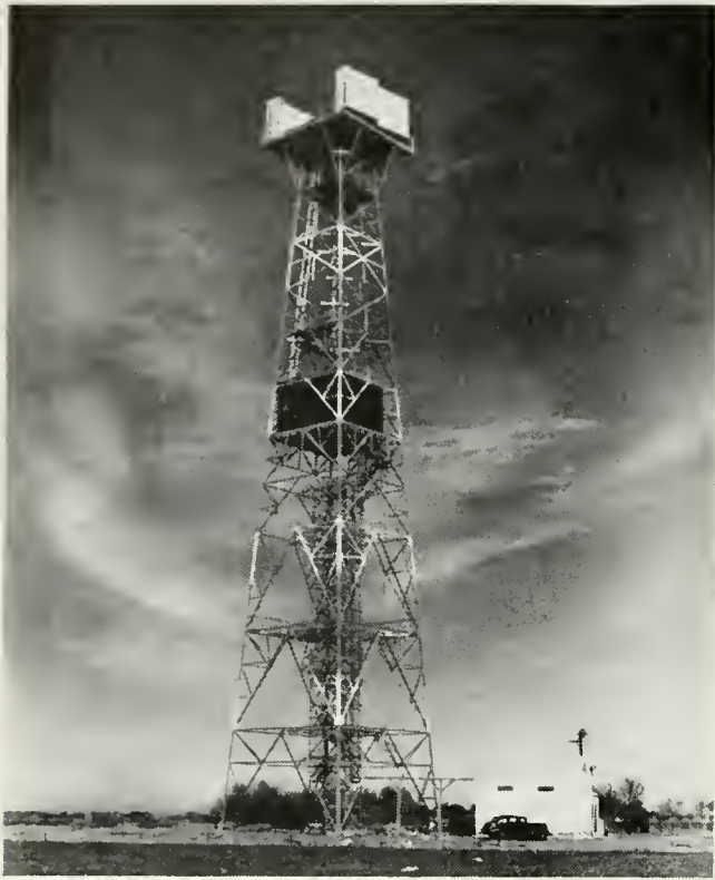
“Cabin in the sky”: on the route between Omaha and Denver several of these towers support transmitting and receiving equipment about 100 feet above ground
