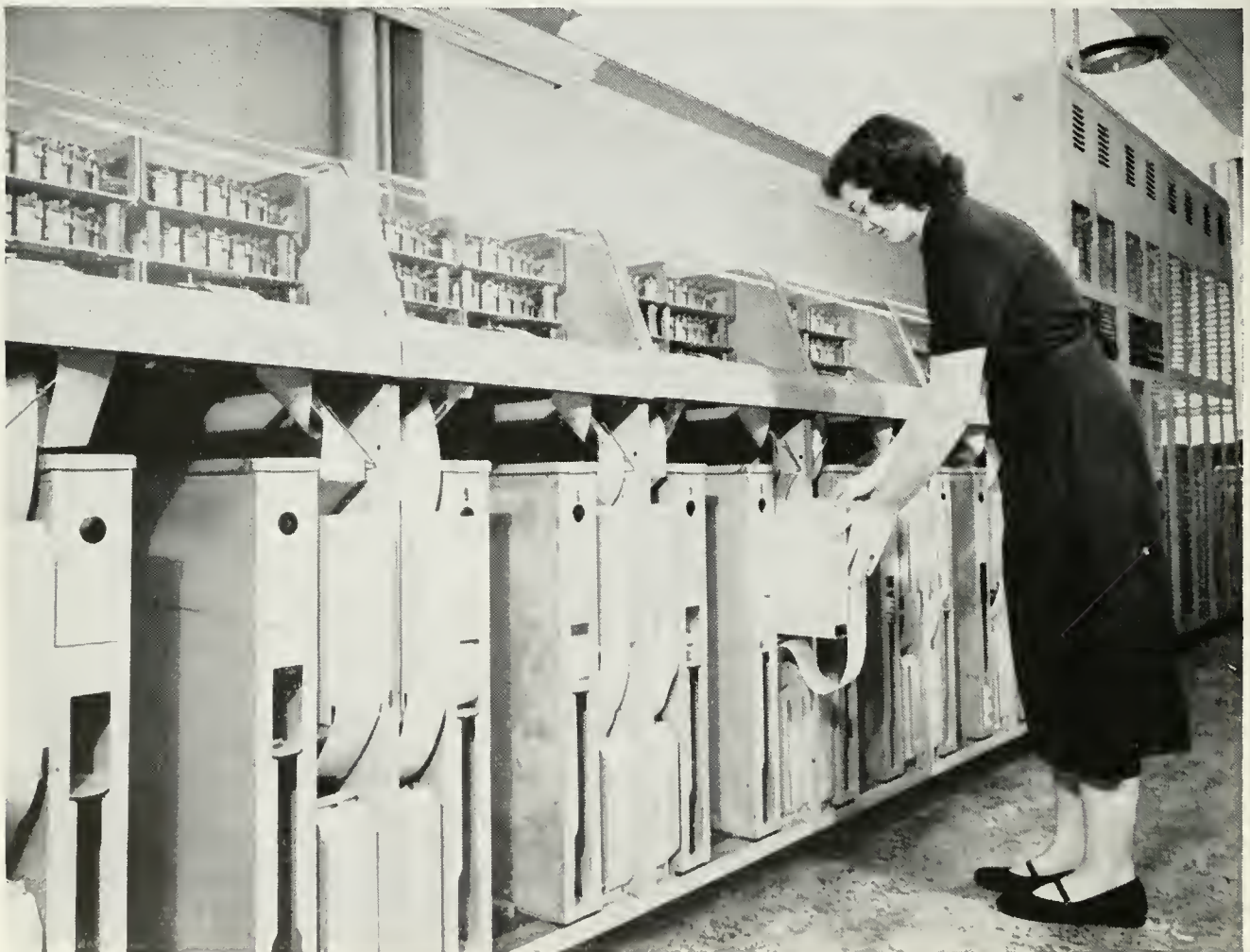
Customer dialing of long distance calls requires automatic equipment to time each call, compute the charge, and record other details necessary for billing. The details of many calls are first recorded electrically on a single tape, which is then unscrambled by this computer, transcribing the data in proper sequence on other tapes
