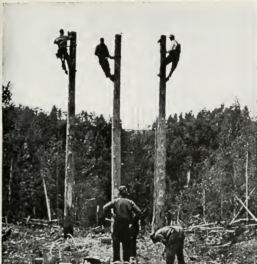
Long span construction makes it up the hill in one jump
