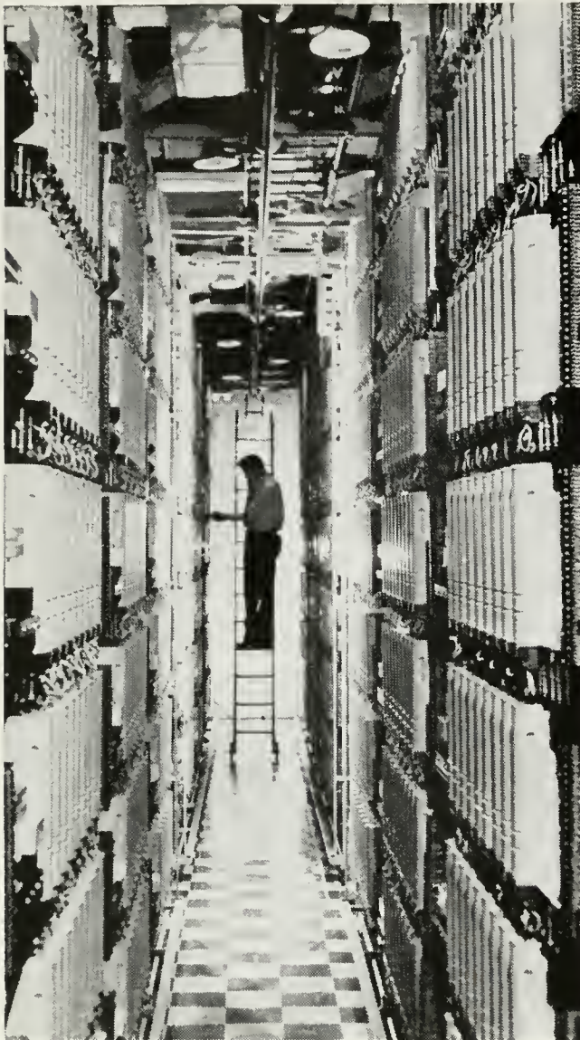
A manual routine testing operation on dial equipment: checking selectors in a step-by-step central office
