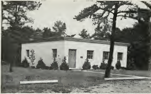
The community dial office at Deer Park, N. Y., is of appropriate design for a small community
