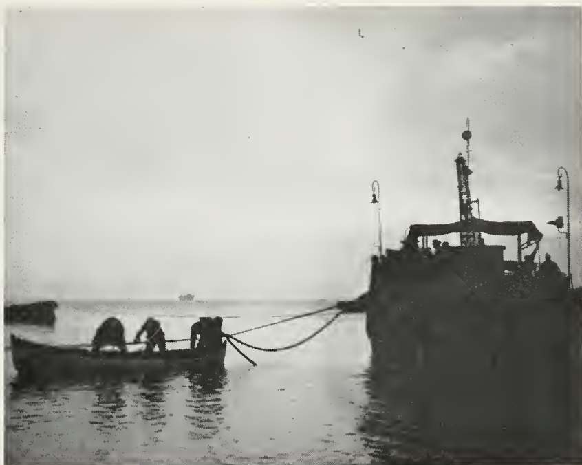
Cables provide new voice paths beneath the historic Bosphorus. Below: The Turkish P. T. T. now handles the laying of its submarine cables
