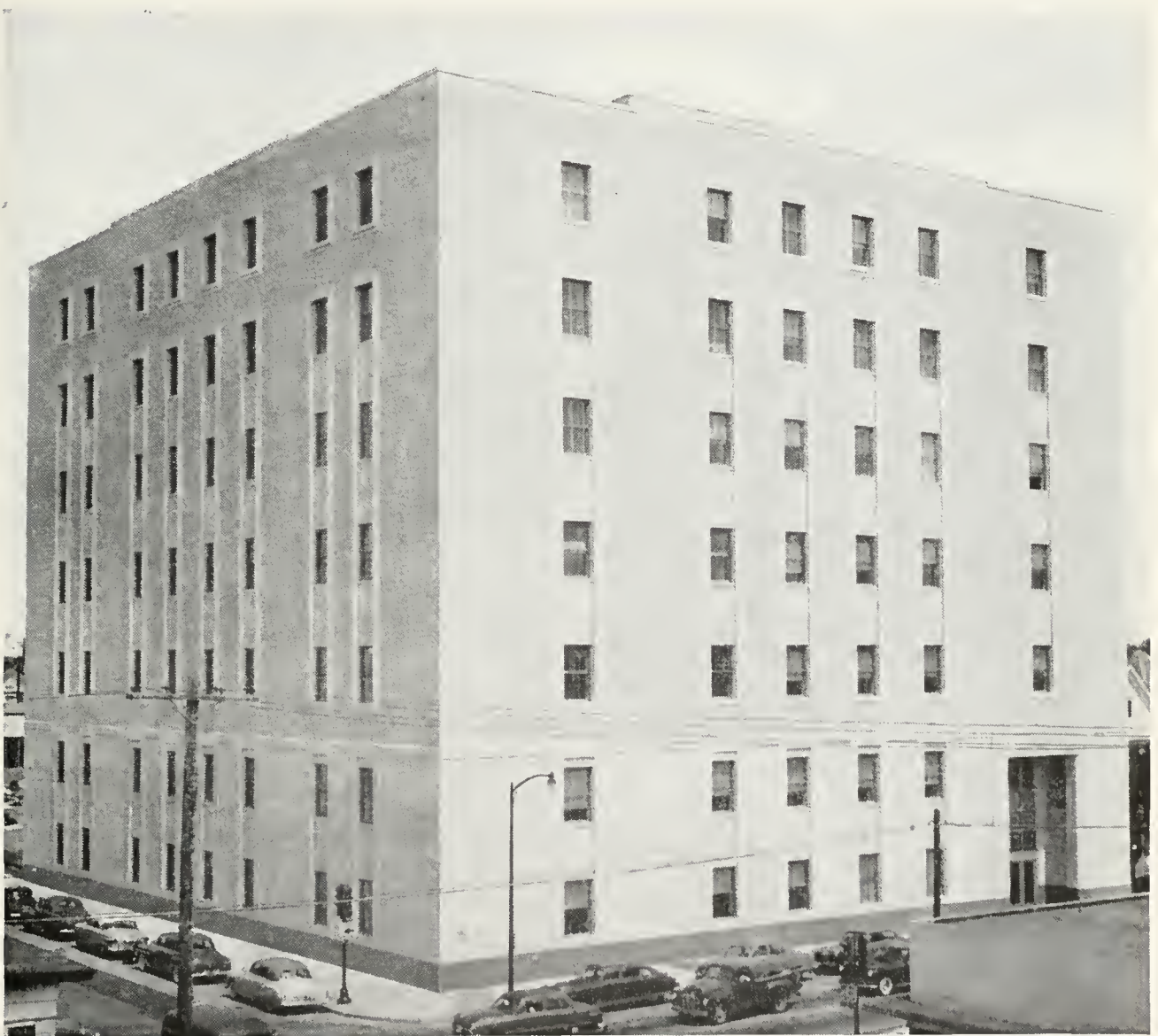
This newly completed building at Houston, Tex., is an example of modern and efficient design for housing the latest type of toll switching equipment
