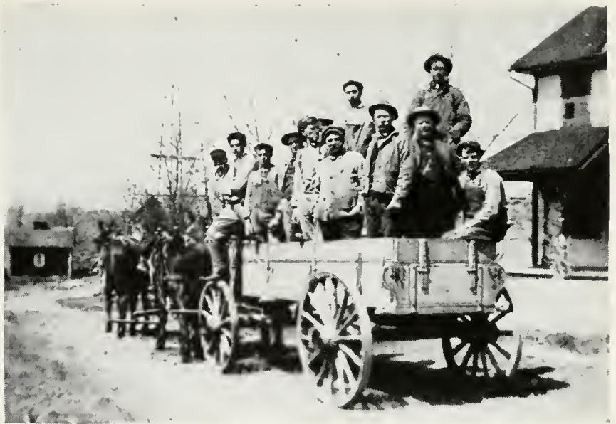
A line crew at Hazelton, Pa., in 1910, all set for a big day's work-out
