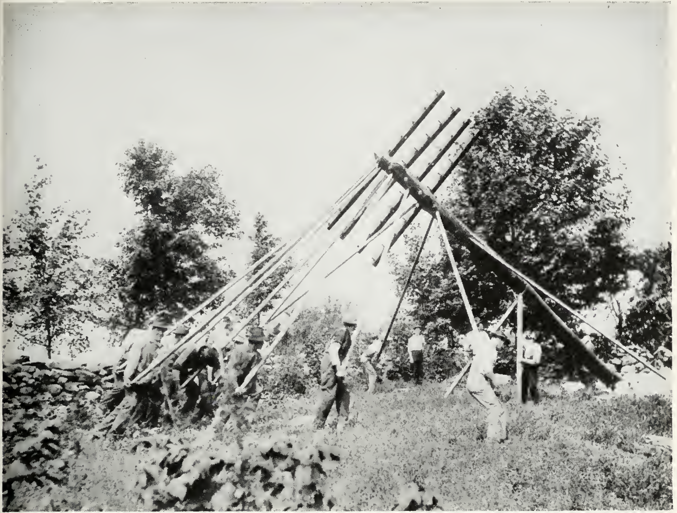
Although the gang evidently raised this 40-foot pole successfully, scarcely a man is piking in accordance with later and safer methods
