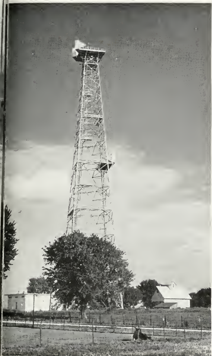
Antennas on different levels are sometimes needed to avoid reflection of signals
