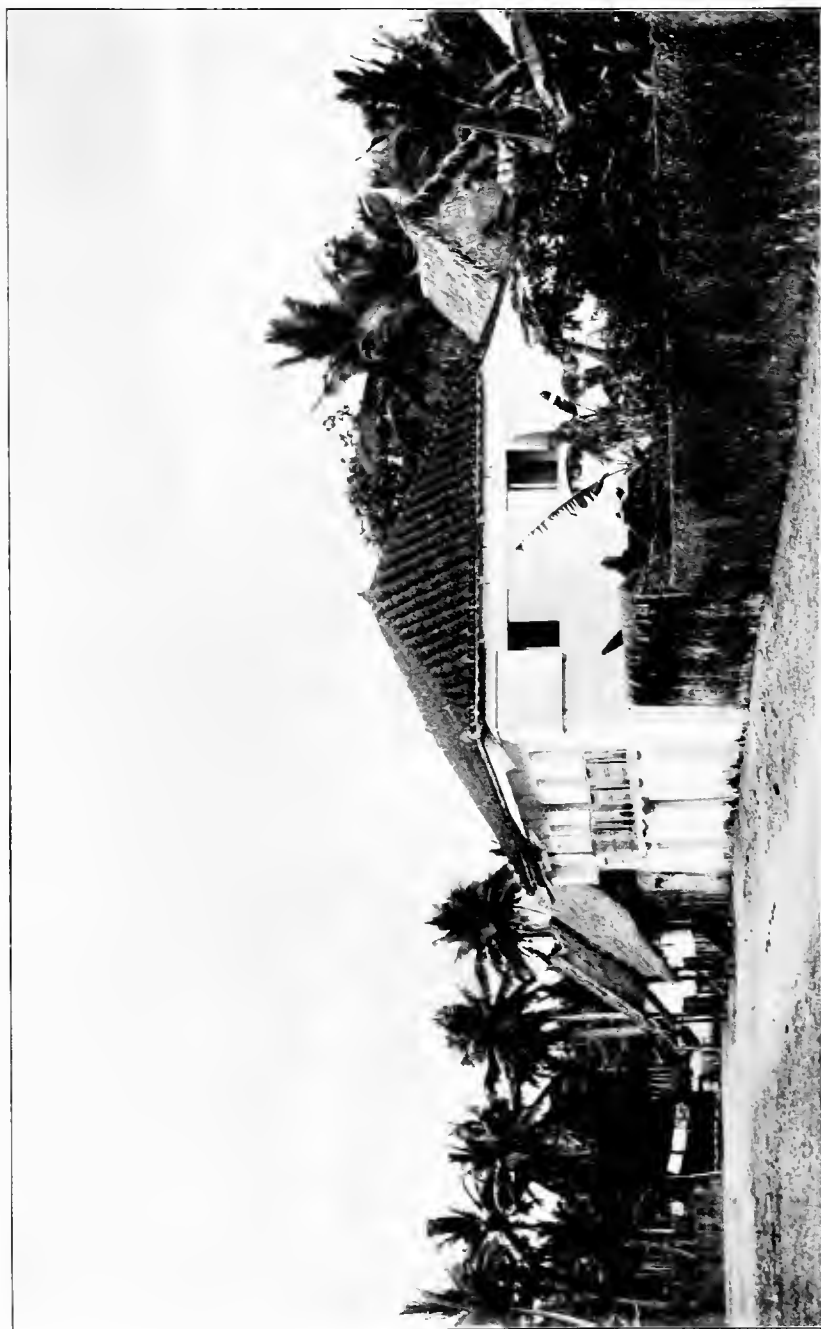
HOUSE WITH THICK WALLS OF MASONRY AND ROOF OF TILES, THATCHED KITCHEN IN REAR, AND GARDEN ENCLOSED BY WALL.
