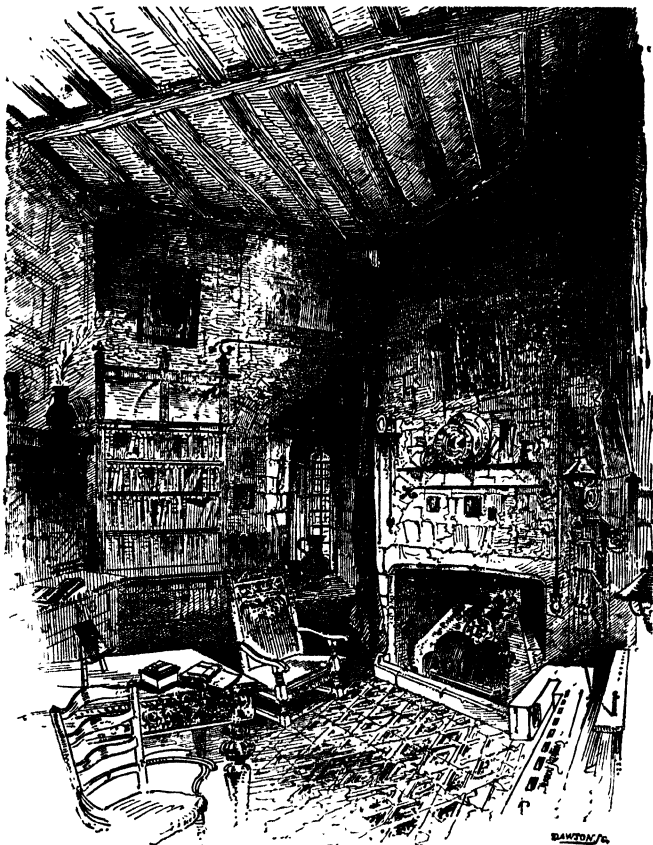
PRISON ROOM ABOVE THE NORMAN TOWER
