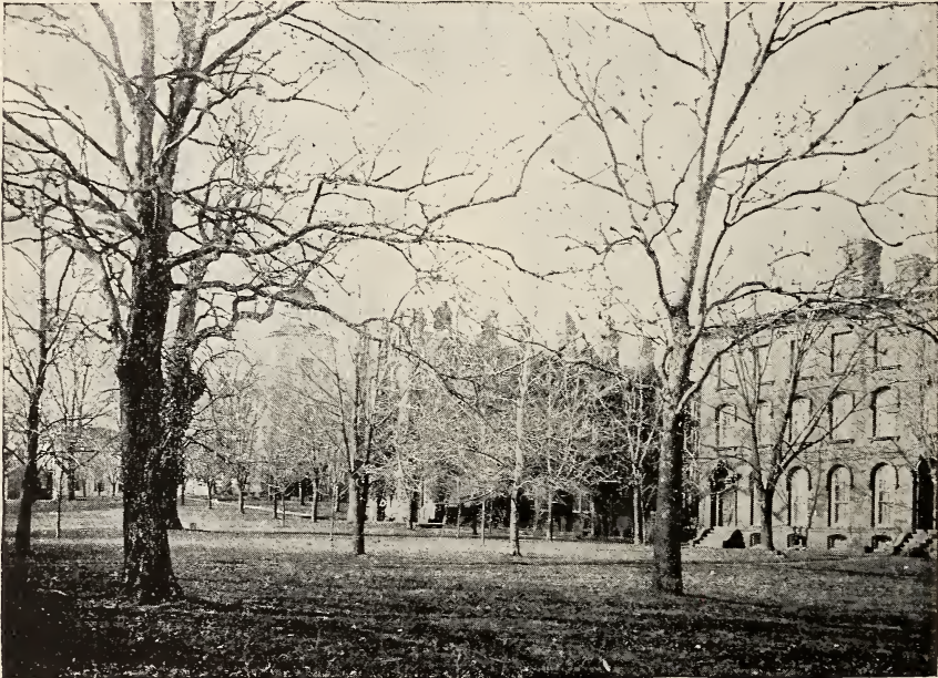
GENERAL VIEW OF ST. JOHN'S COLLEGE, ANNAPOLIS, MD.
