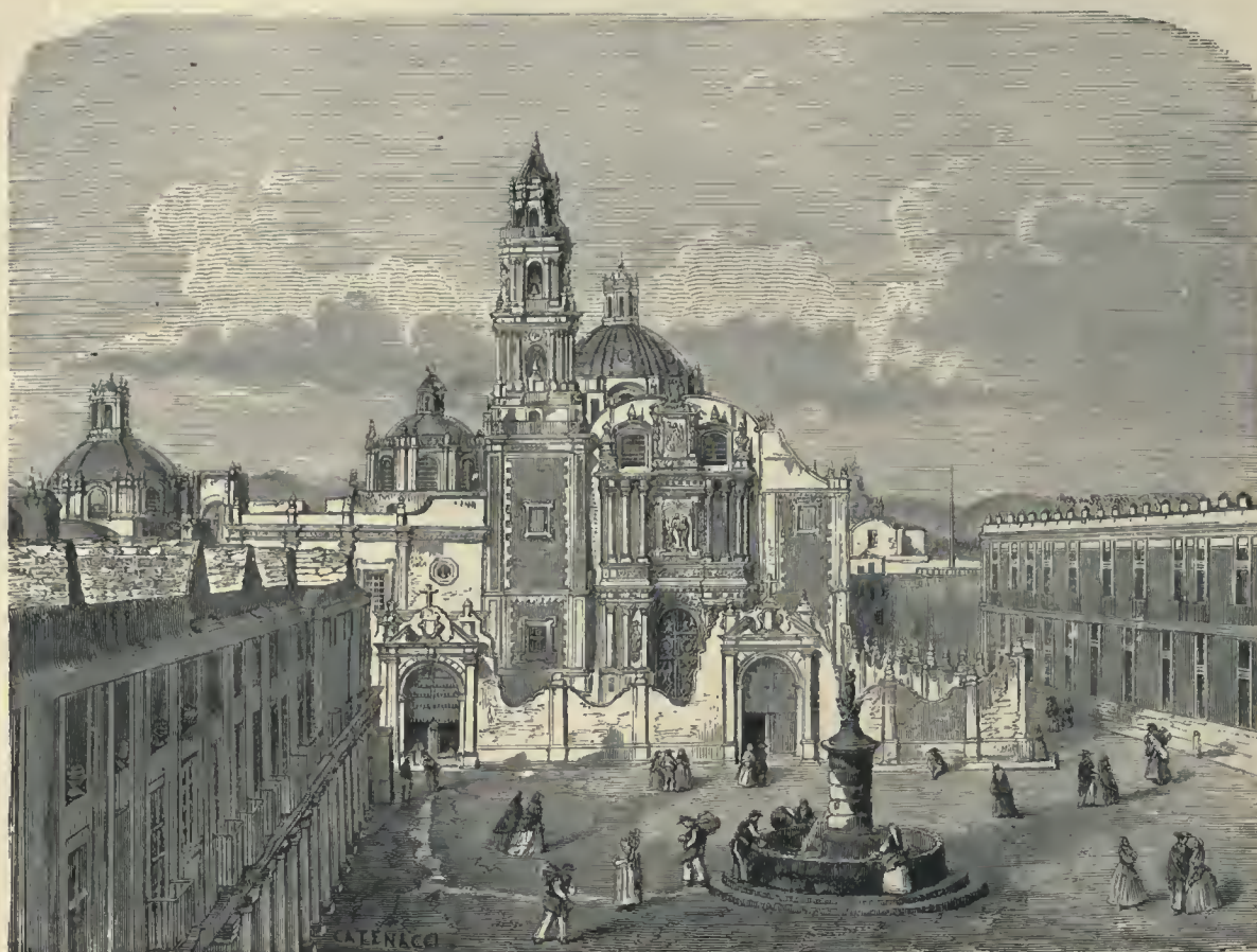
Church and Square of San Domingo, City of Mexico.
