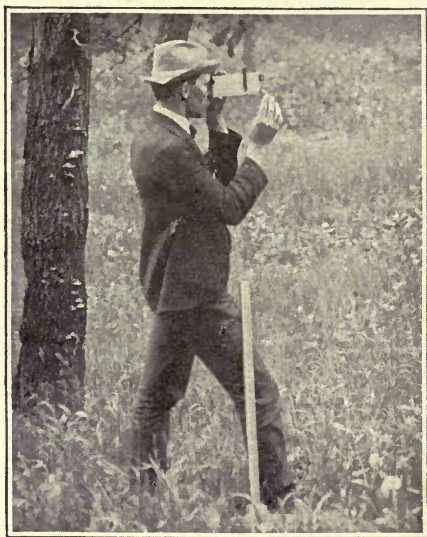
FIG. 65.—The mirror hypsometer in use.
