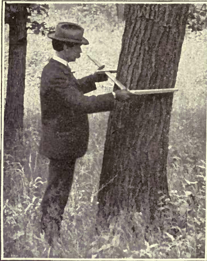
FIG. 63.—Calipering a tree.
