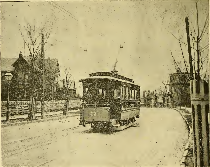
DAFT ELECTRIC ROAD, CINCINNATI, ROUNDING CURVES.
