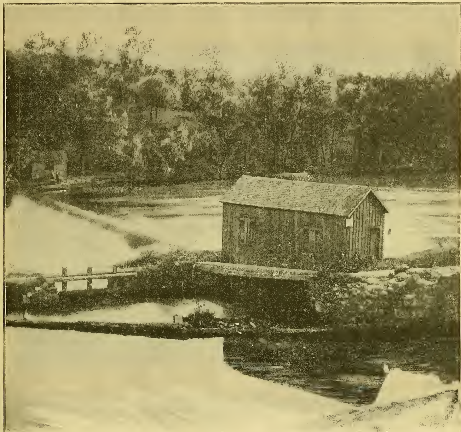
THE ROCK WAY RIVER AT THE BOONTON FALLS, SHOWING INTAKE OF THE MORRIS CANAL (ELEVATION ABOVE TIDE-WATER ABOUT 560 FEET).
