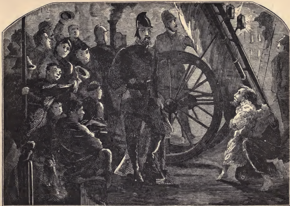
THE FIRE ESCAPE.
