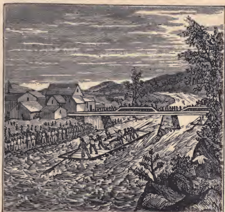
SHOOTING THE BRIDGE.
