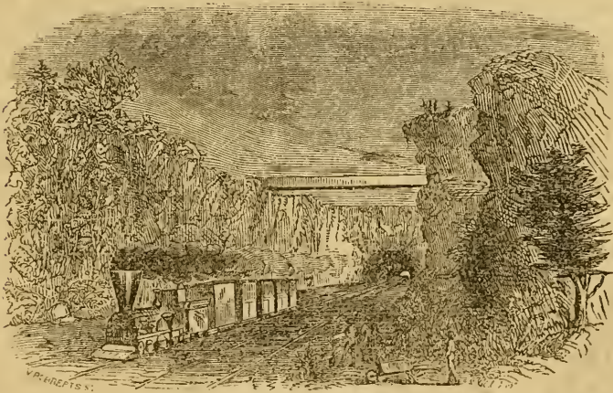
Tunnel at New Hamburg.
