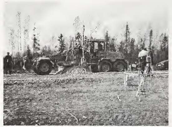
Figure 6: The site tests of the 3-D blade control system.
