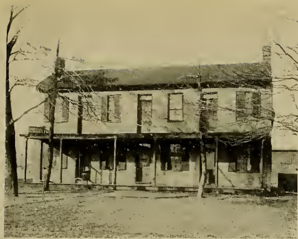
OLD PENNSYLVANIA HOUSE, SPRINGFIELD
