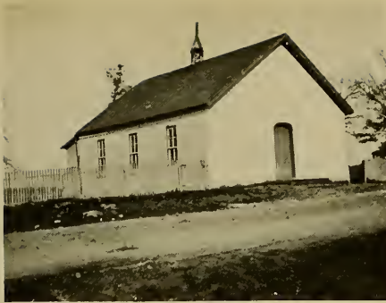
SINKING CREEK CHURCH, SPRINGFIELD TOWNSHIP
