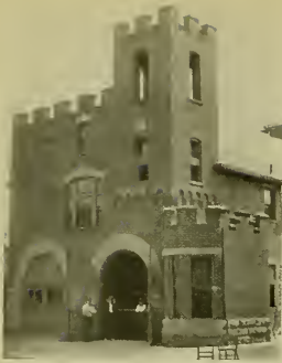
FACTORY STREET ENGINE HOUSE, SPRINGFIELD
