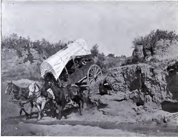
A Bates' Hole Road
